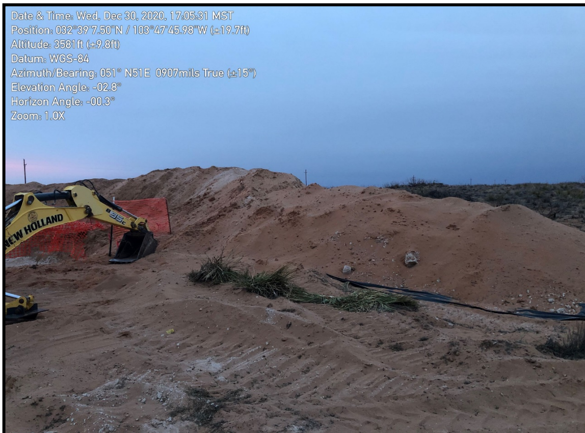
View of STP-4 during excavation activities, facing northeast.
