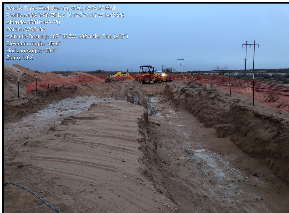
View of Reclamation Soil Excavation area during excavation activities, facing south.
