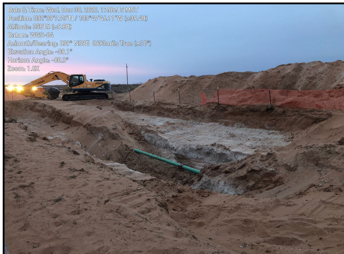
View of entire excavation site during excavation activities, facing northeast.
