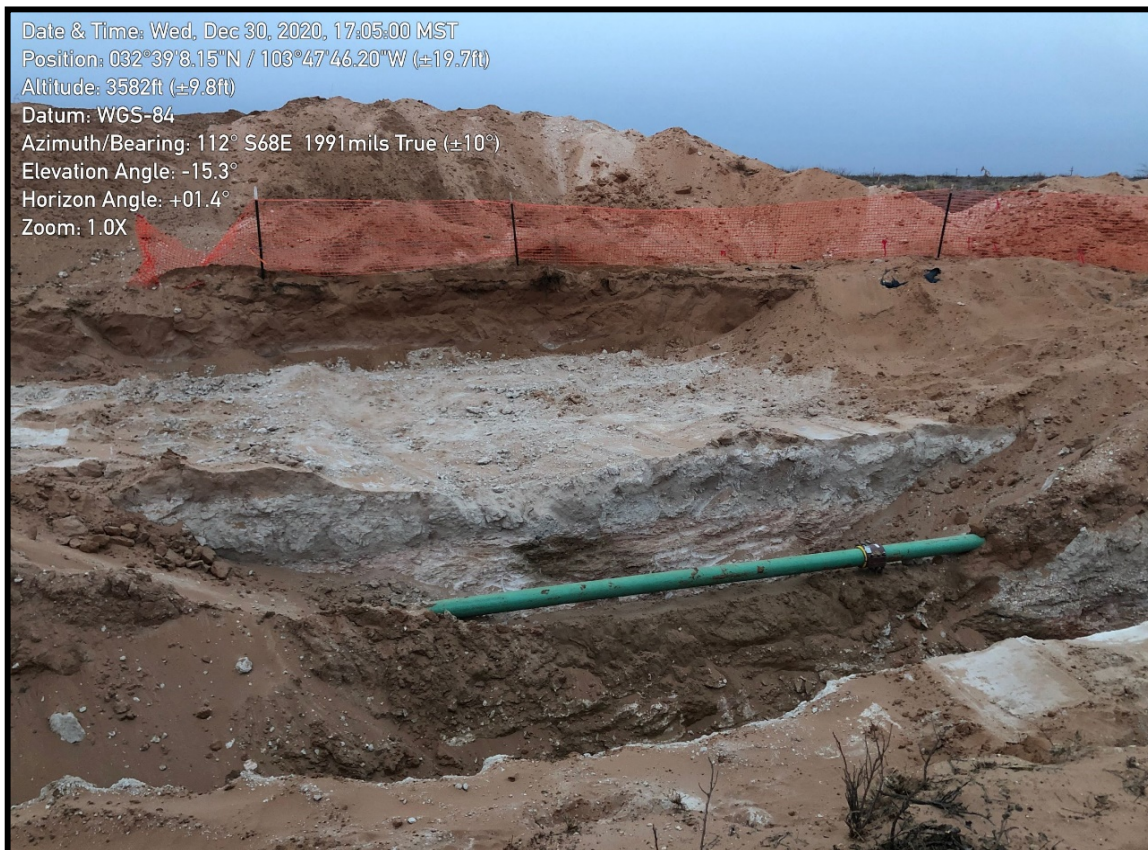
View of pipeline with clamp during excavation activities, facing southeast.
