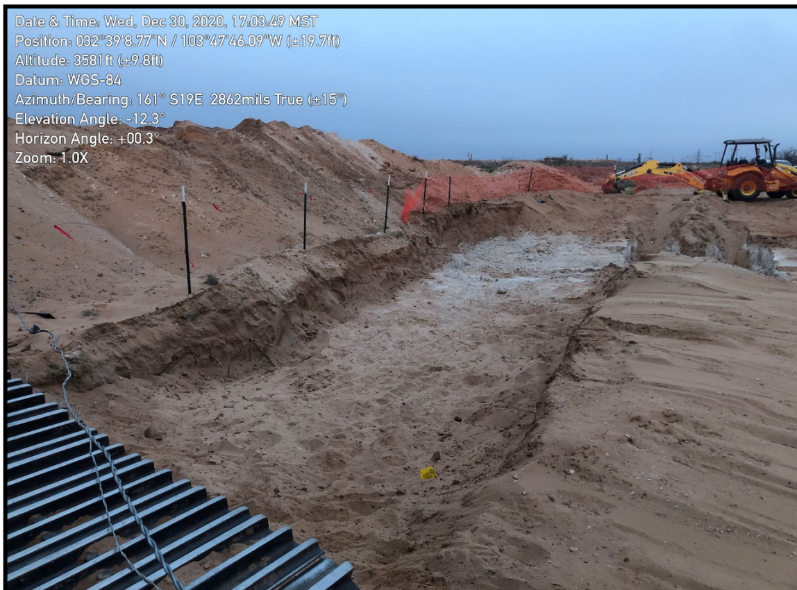
View of Reclamation Soil Excavation area during excavation activities, facing southeast.
