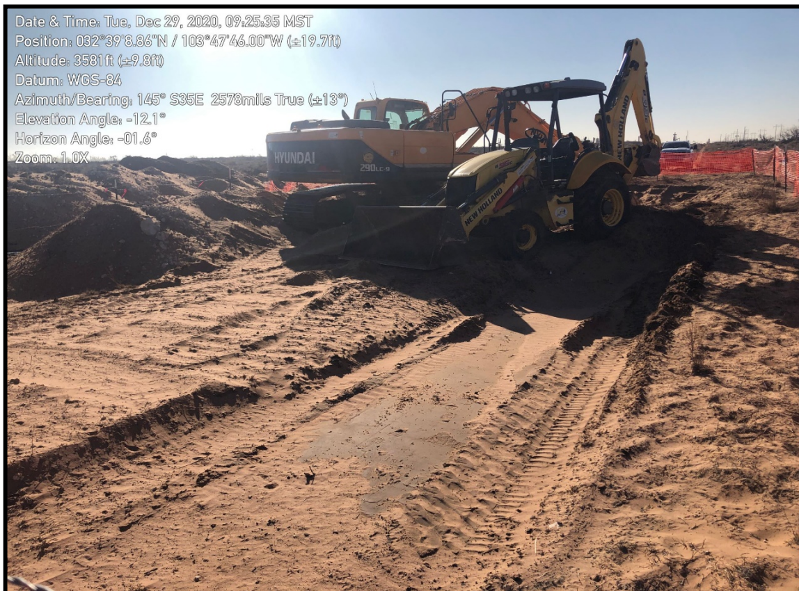
View of surficial staining during excavation activities, facing southeast.
