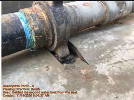
Viewing Direction: South
