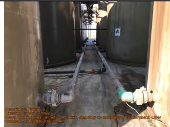
Viewing Direction: West
