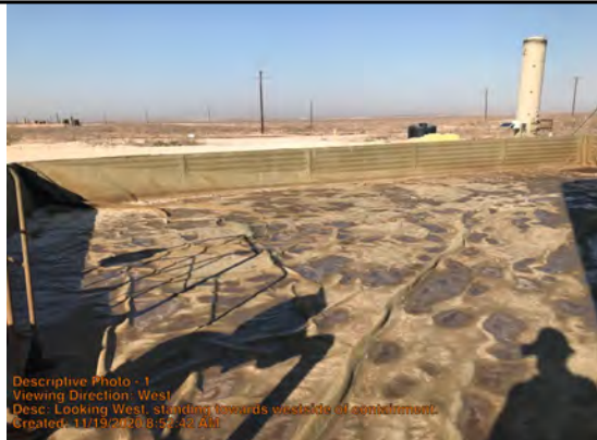
Viewing Direction: West
