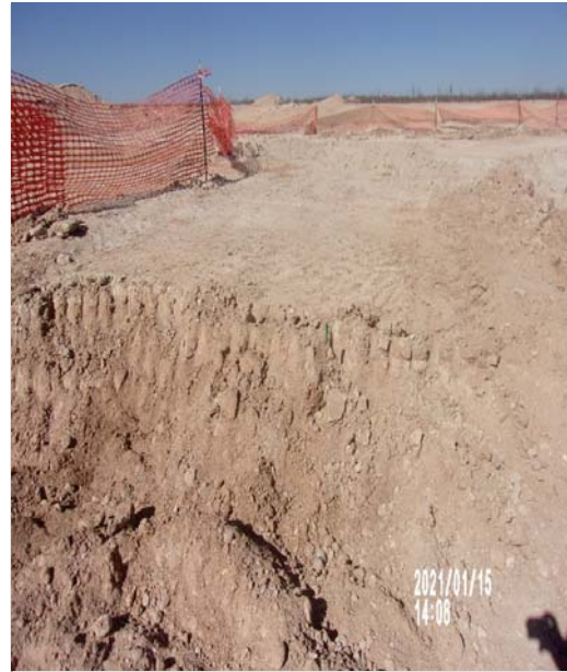
View South – Sidewall sample location (dark green flag) 20.
