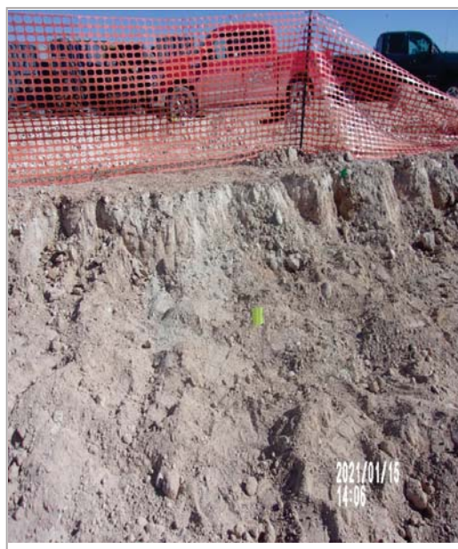
View East – Confirmation sample location (lime green flag) 26 and Sidewall sample location (dark green flag) 14.
