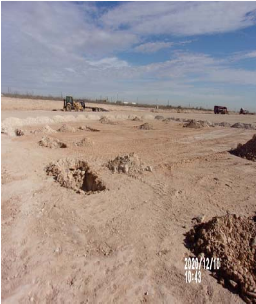
View Northeast – Delineation sample locations within the release footprint (i.e., Auger Holes 1 thru 10).
