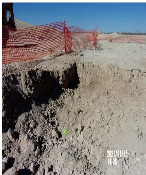
View North – Confirmation sample location (lime green flag) 31 and Sidewall sample locations (dark green flag) 19 and 20.
