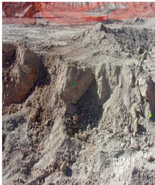
View West – Confirmation sample location 19 (lime green flag) and Sidewall sample locations (dark green flag) 23 and 24.
