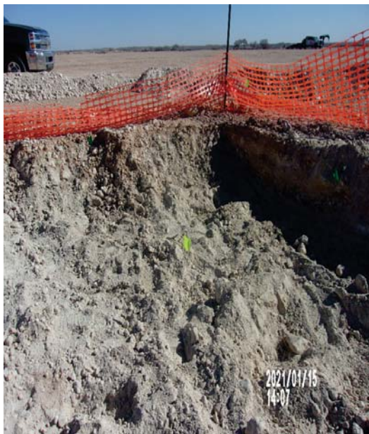
View Southeast – Confirmation sample location (lime green flag) 31 and Sidewall sample locations (dark green flag) 18 and 19.
