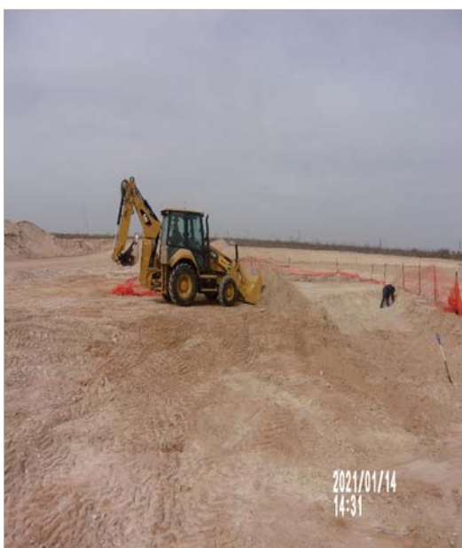
View North – Excavation of impacted material ongoing.
