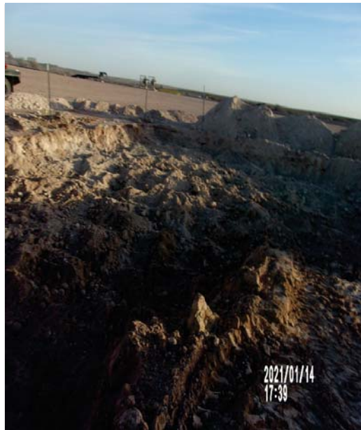
View Southeast – Excavation of impacted material ongoing.
