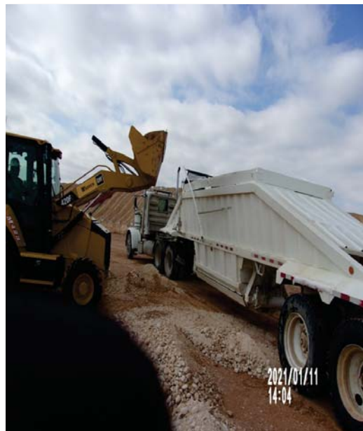
View Southwest – Impacted material excavated to 2 ft bgs being exported offsite to a Cimarex approved disposal.
