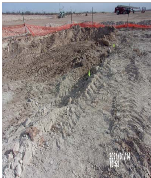
View Northeast – Confirmation sample locations (lime green flags) 1, 2, 6, 7, 8, and 9.
