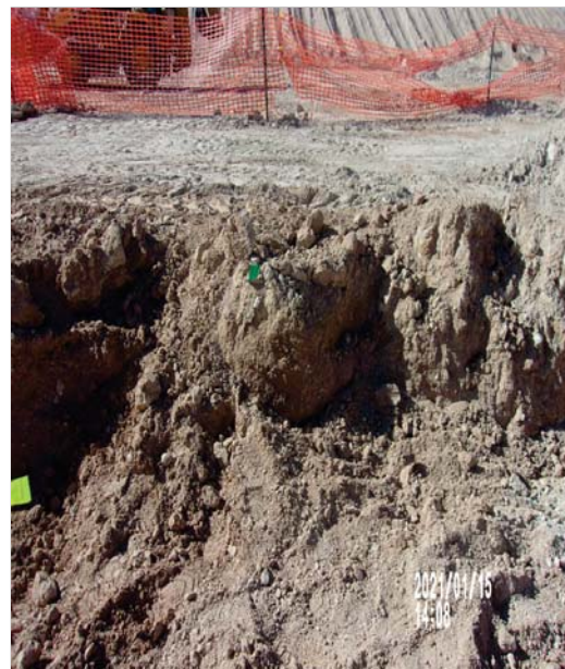
View South – Sidewall sample location (dark green flag) 22.
