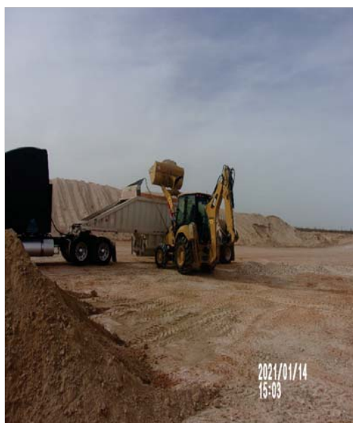
View Northwest – Excavated impacted material being loaded for export offsite to a Cimarex approved disposal.
