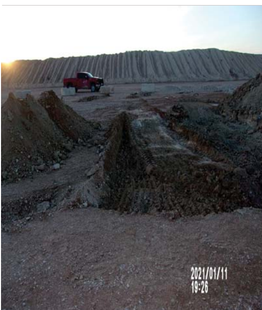
View West – Impacted material excavated to 2 ft bgs to be exported offsite to a Cimarex approved disposal.
