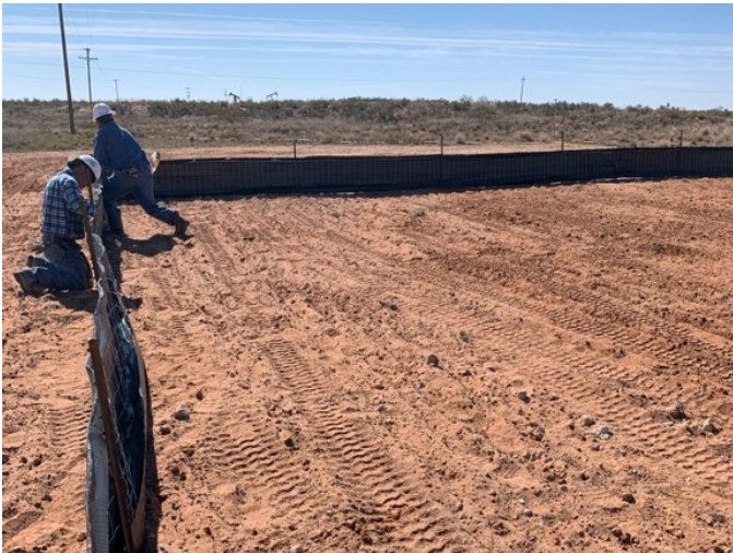
Installing silt net fencing, facing southwest
