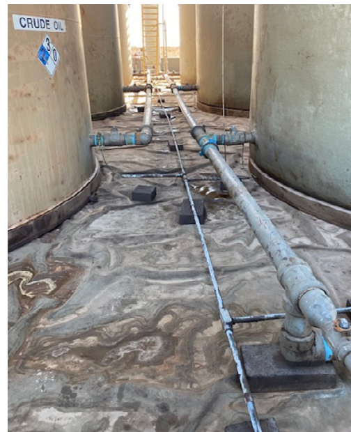
Picture 8- East face, west edge of containment 10-Mar
