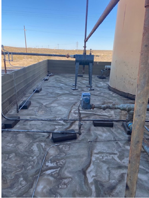
Picture 9- North face, southwest edge of containment 10-Mar
