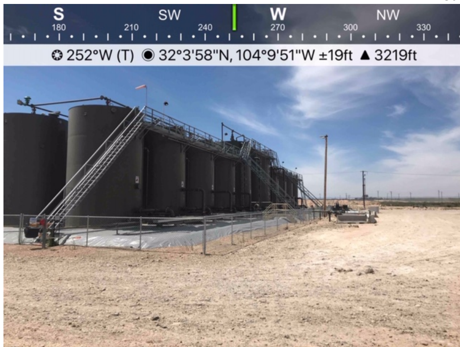
Spill within lined containment viewing southwest/west
