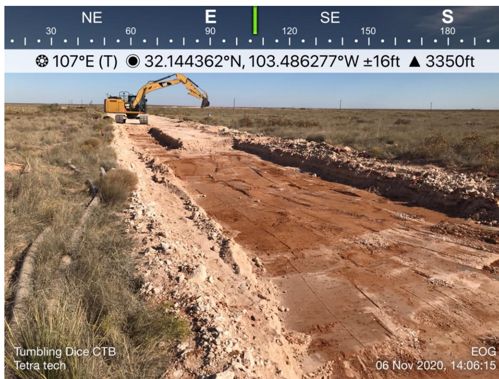
View East, areas of Bottom Holes (7-17)
