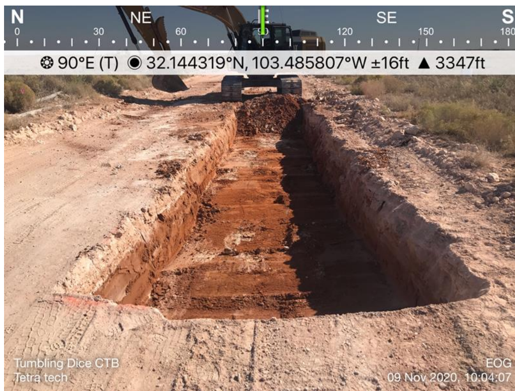
View East, areas of Bottom Holes (1-3)
