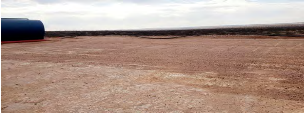
Figure 1: Graded area shows the western half of the release extent that was removed and replaced with clean caliche. Frac tanks are visible photo left. Photo is viewing south-southeast. GPS: 32.4158530 N, -103.6036710 W. Date/Time: 2019-02-08 09:28:16
