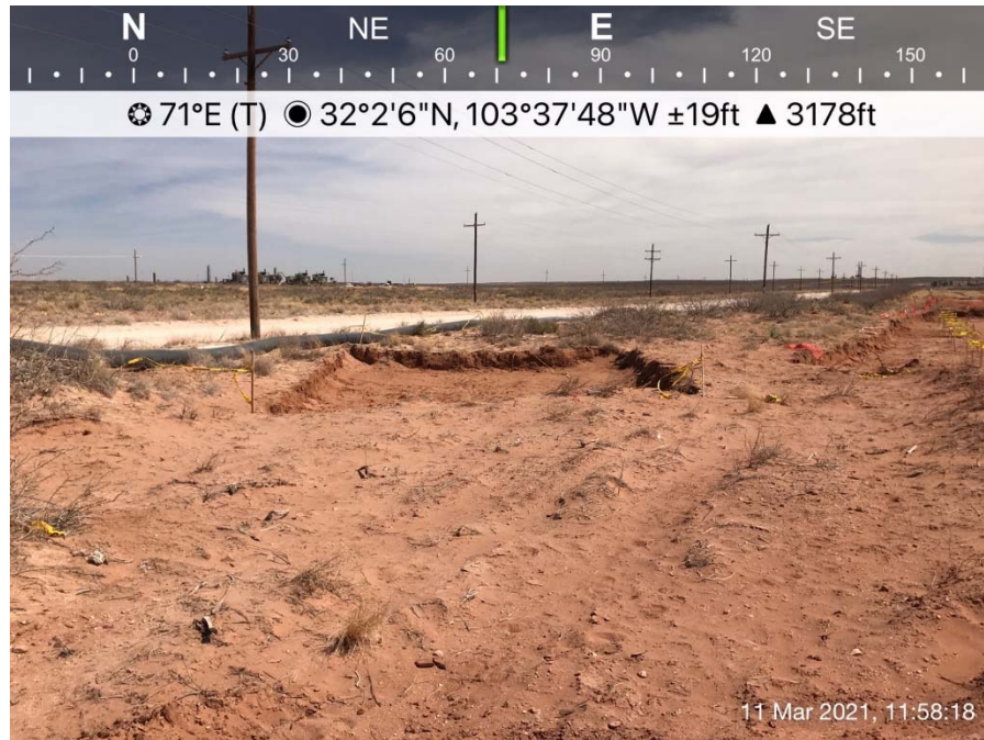
Photograph of Area 1, excavated to 1-foot bgs, March 11, 2021.
