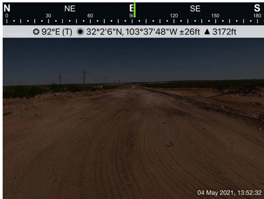
Photograph showing Area 2, backfilled and seeded, May 4, 2021.
