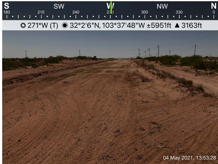
Photograph showing Area 2 and Area 3 backfilled and seeded, May 4, 2021.
