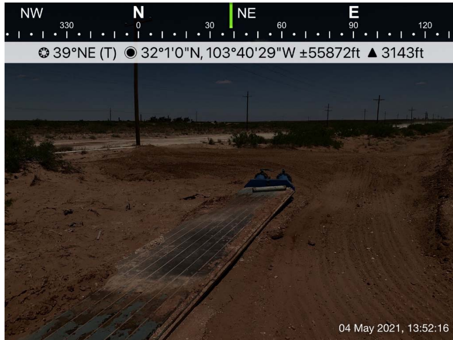
Photograph showing Area 1 backfilled and seeded, May 4, 2021.
