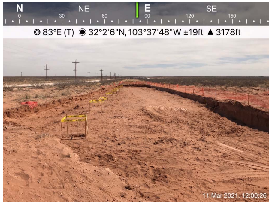
Photograph of Area 2, excavated to 3 feet bgs, viewing to the east, March 11, 2021.
