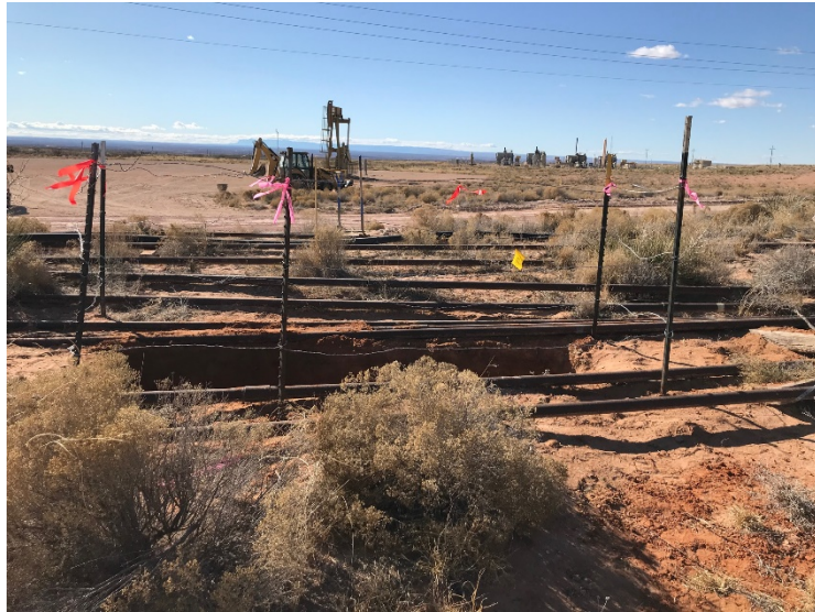
Photograph 1: South facing view of the excavation.
