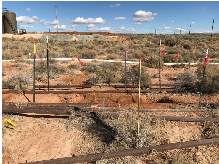
Photograph 3: North facing view of the excavation.
