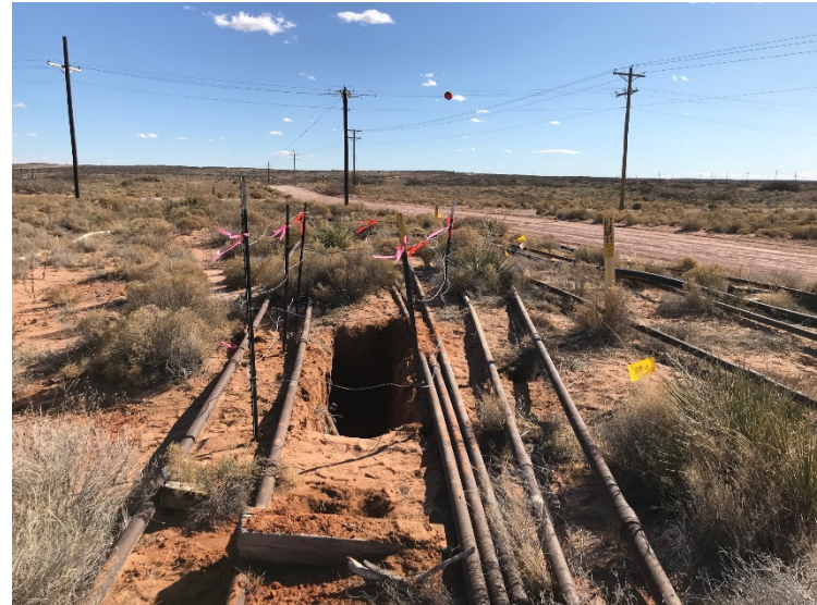
Photograph 2: Southeast facing view of the excavation.
