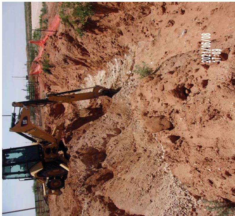
View West – Remediation activities (excavation of impacted material) ongoing adjacent to and around sample locations Bottom Hole 11 and Bottom Hole 13.
