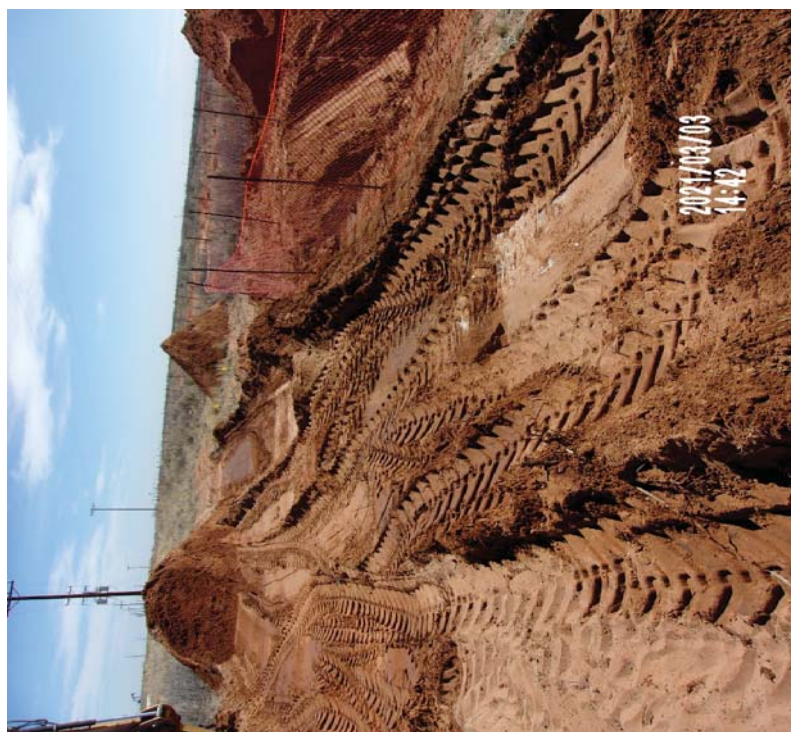
View East – Remediation activities (surface scrape of impacted material within the release footprint) ongoing.
