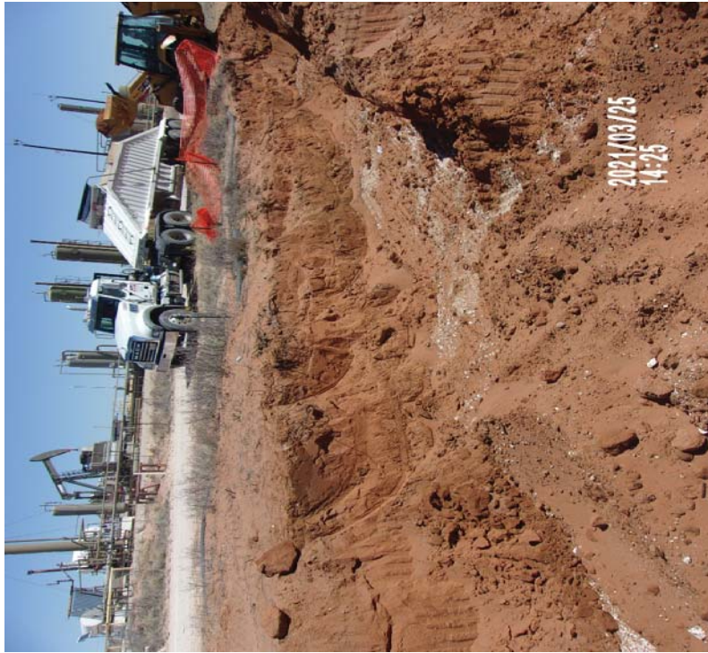
View Northeast – Remediation activities (excavation of impacted material within the release footprint) ongoing. Material was transported to an approved disposal facility.
