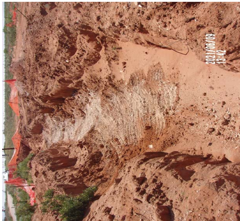
View East – Remediation activities (excavation of impacted material) ongoing adjacent to and around sample location Bottom Hole 7.
