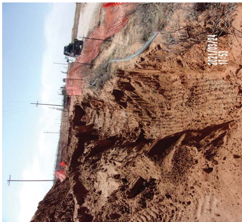
View West – Remediation activities (excavation of impacted material within the release footprint) ongoing.
