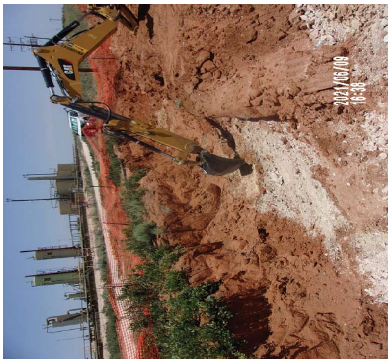
View Northeast – Remediation activities (excavation of impacted material) ongoing adjacent to and around sample location Bottom Hole 16.
