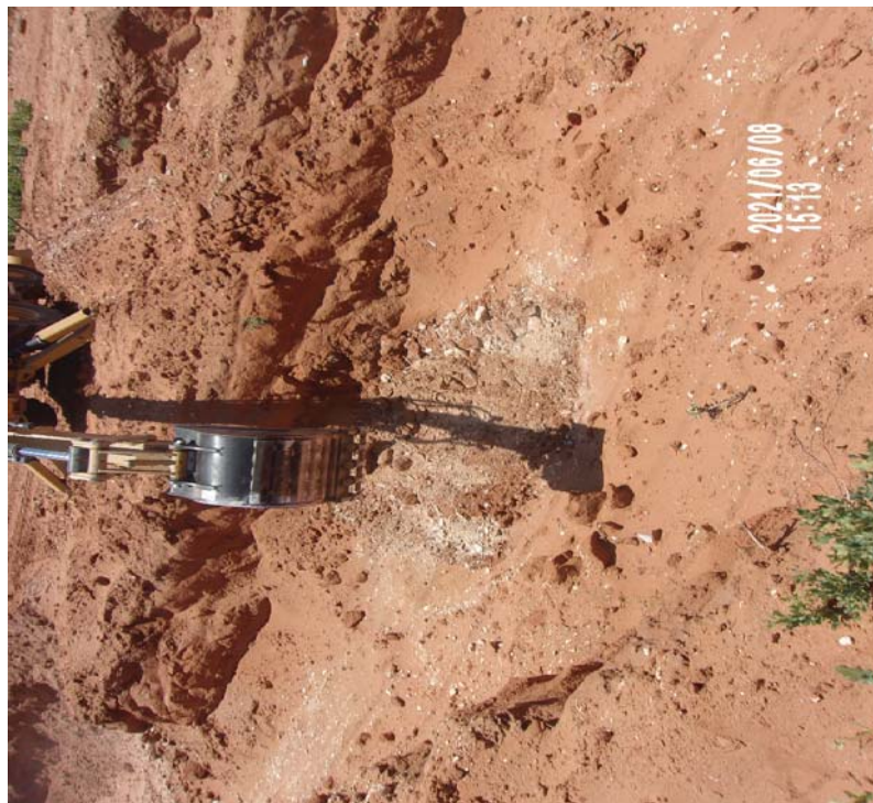
View South – Remediation activities (excavation of impacted material) ongoing adjacent to and around sample location Bottom Hole 10.
