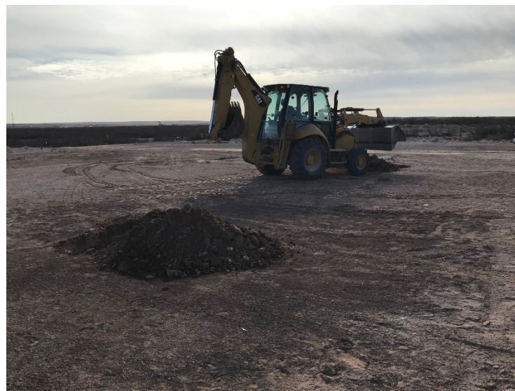
Photograph 2: Southeast facing view of stained area during potholing activities.
