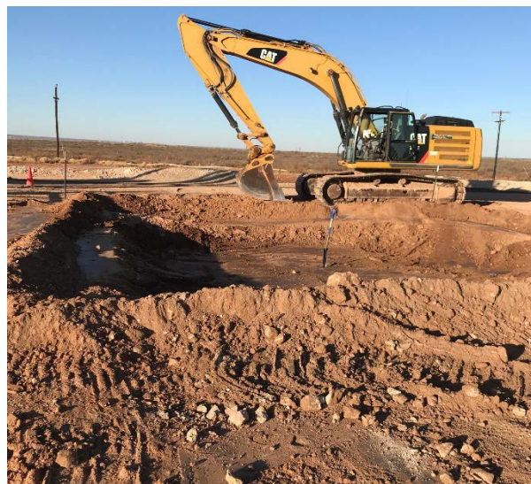
Photograph 4: North facing view of open excavation.
