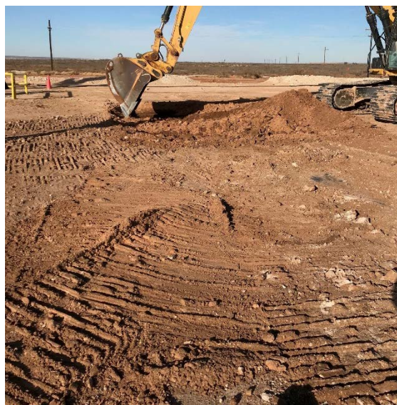
Photograph 3: North facing view during excavation activities.
