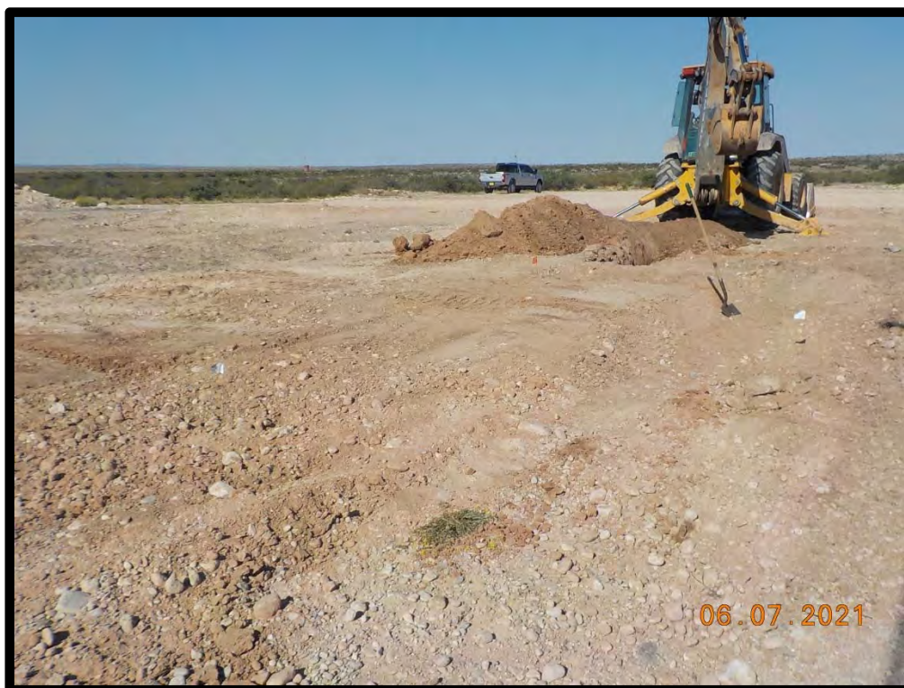
PHOTOGRAPH NO. 6 – A view collected during the additional assessment activities on June 7, 2021. The view is towards the southwest.
