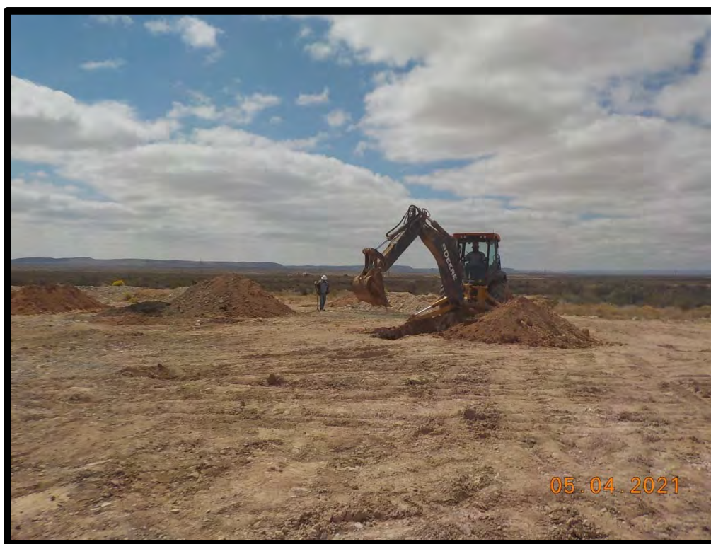
PHOTOGRAPH NO. 4 – A view collected during the installation of test excavation SP-W on May 4, 2021. Sample location SP-1.A can be seen in the left side of the photograph. The view is towards the south.
