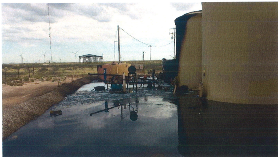
Photo of Release contained in earthen berm. No staining is observed outside of the earthen berm. Photo Date: 9/1/2019
