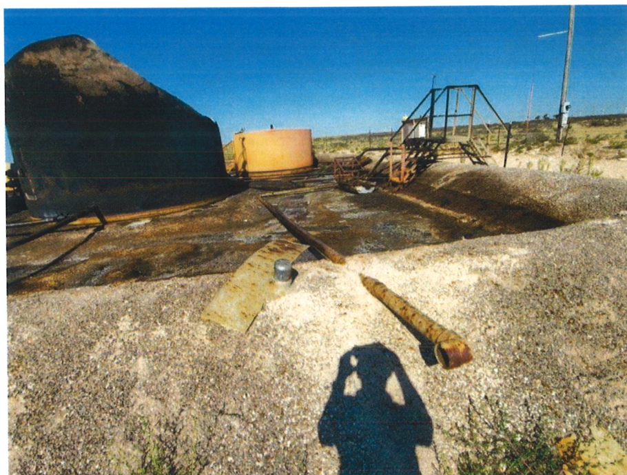
Photo of lined earthen berm after fluids were removed. No staining is observed outside of the earthen berm. Photo Date: 9/3/2019
