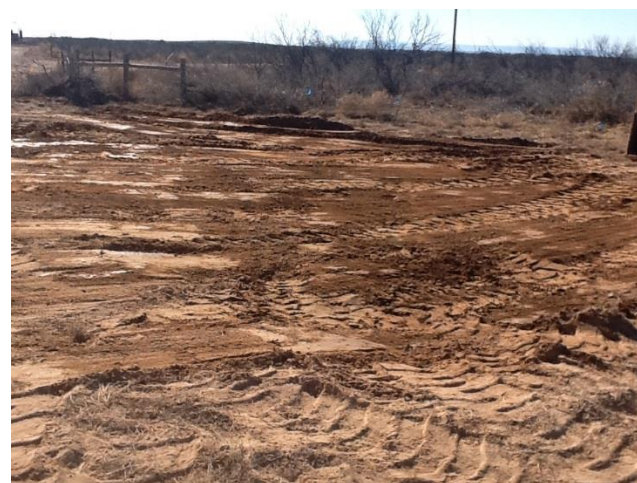
Test Trench restored to grade
