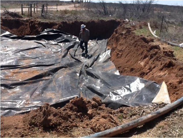
3-16-16 Liner Installation
