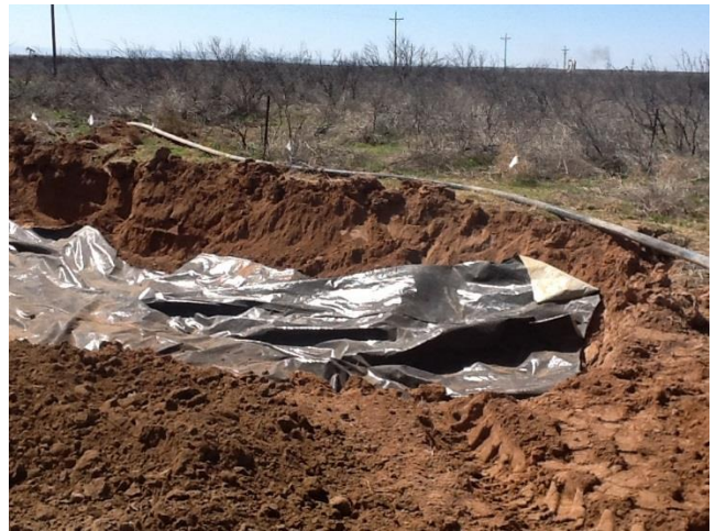
3-17-16 Backfill-unobstructed flowline
