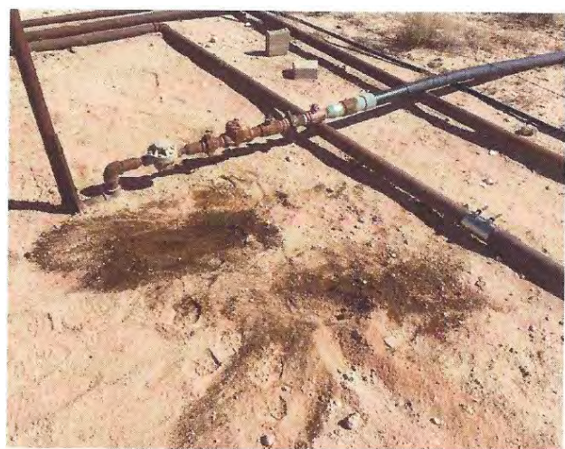
Release by heater treater, scraped top layer by previous slide to show extent of release.
