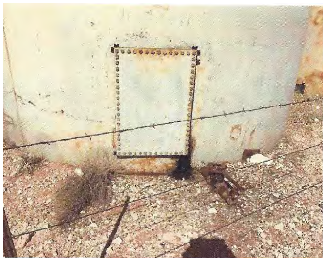
Crude oil tank with leak on manhole cover.
