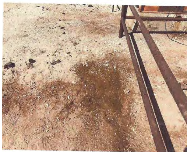
More extensive scuffing of top layer by well-head.
