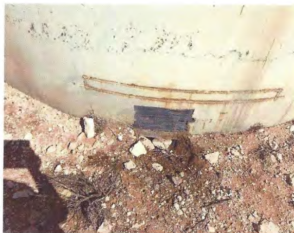
Repair to crude oil tank with duct tape. Release by repair.
