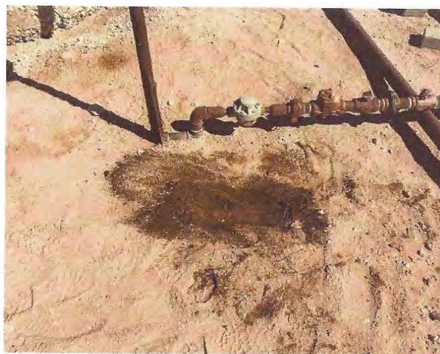
Release by heater treater covered with sand.
