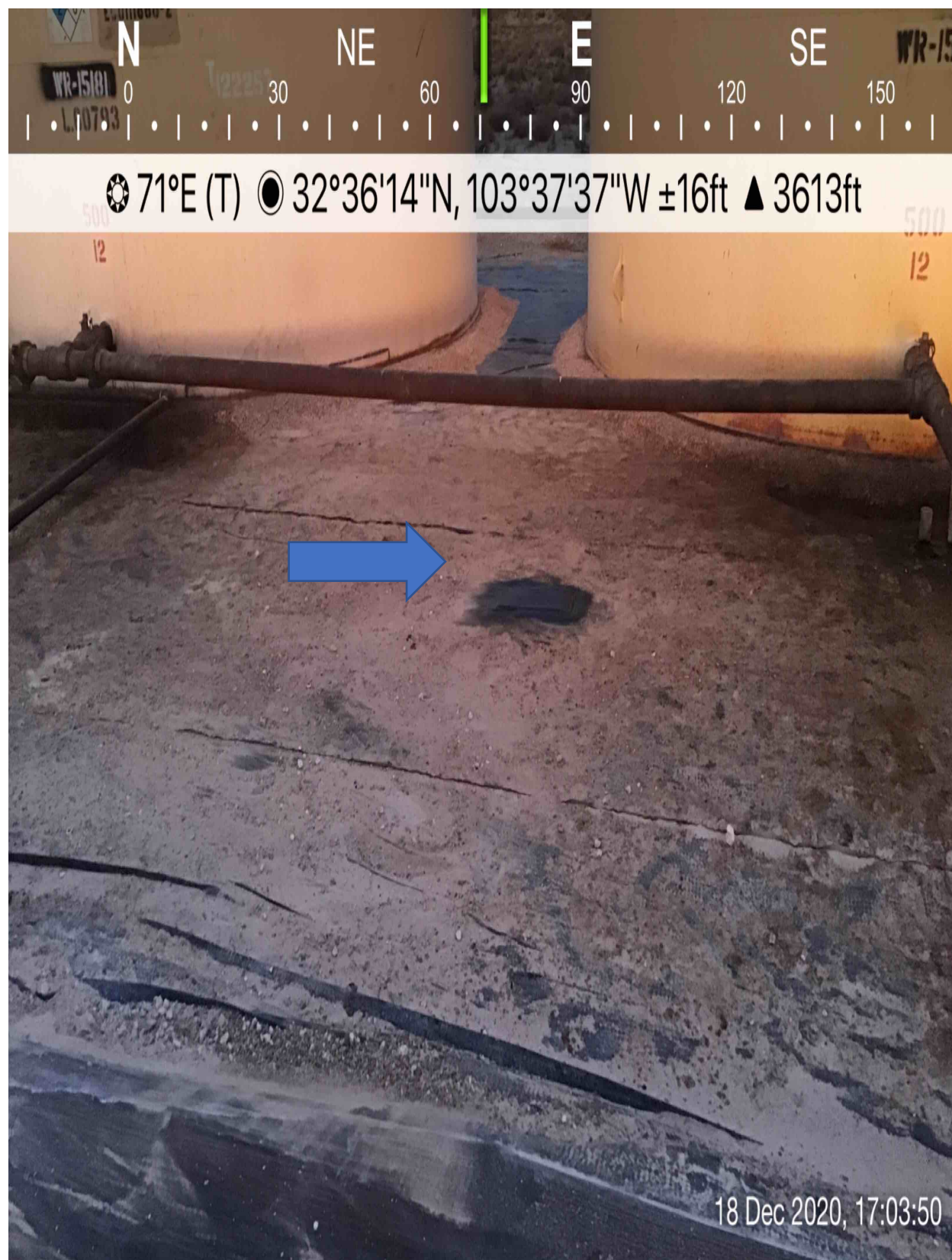
This is the repair to the baseball sized hole in the liner. Looking east northeast.
