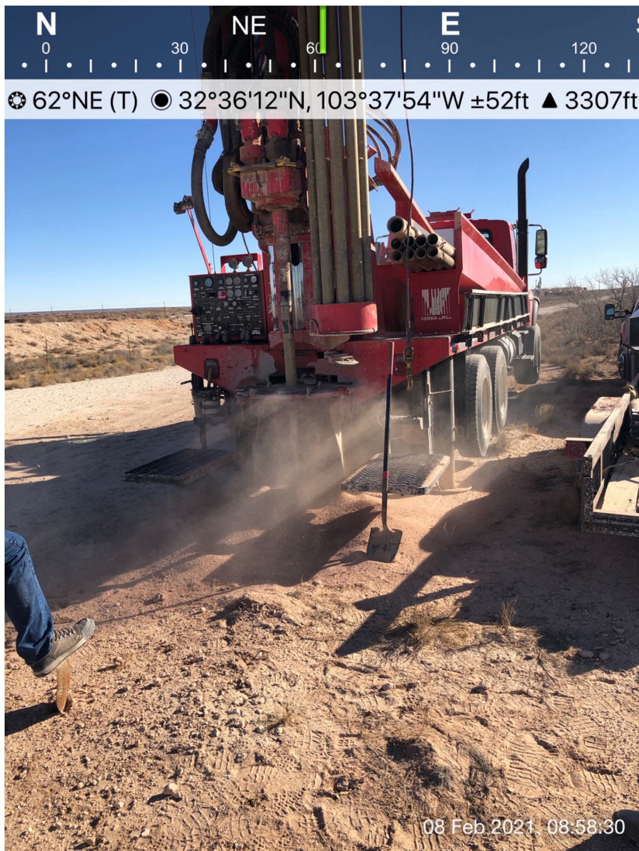
Drilling BH-01: CP-1865 POD 1 using Versa-Drill® V-100NG Air Rotary rig.
