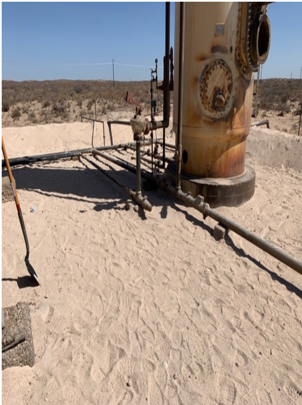
Protective Backfill at the Heater Treater at the South End of the Battery
