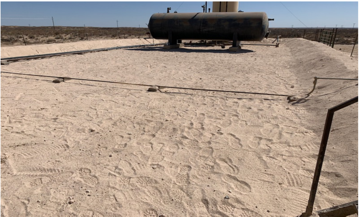
Protective Backfill at the Southern End of the BTA Gem 11-H Battery
