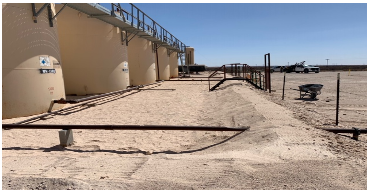
Protective Backfill Cover for the West Side of BTA Gem 11-H Battery Looking South.
