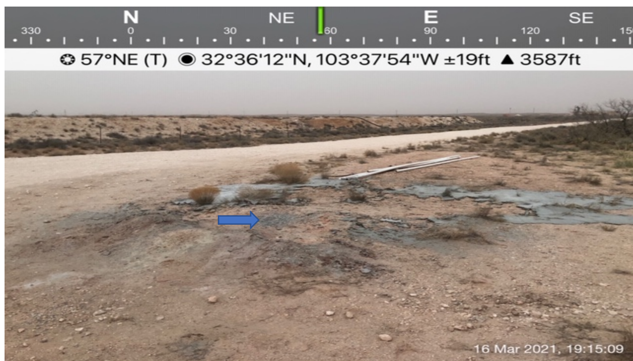
Plugged boring BH-010: CP-1865 POD 1 Dry Hole to 105 feet.
