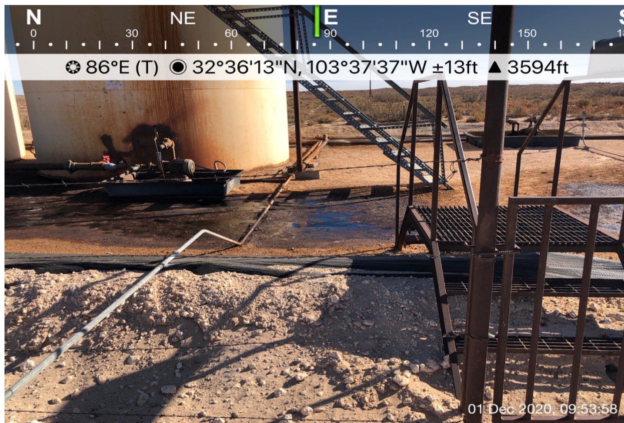
Crude oil and produced water migrated northerly along the western side of the tank battery. Looking nearly due east.
