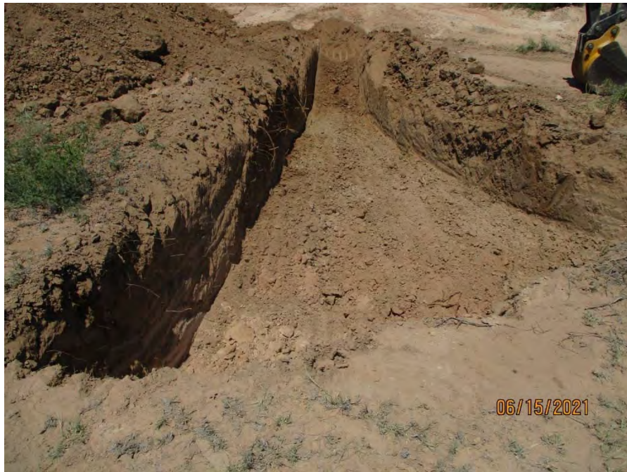
View of Excavation 1 area on June 15, 2021.
