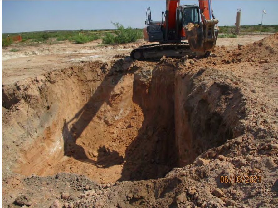
Typical view of the site excavation process.
