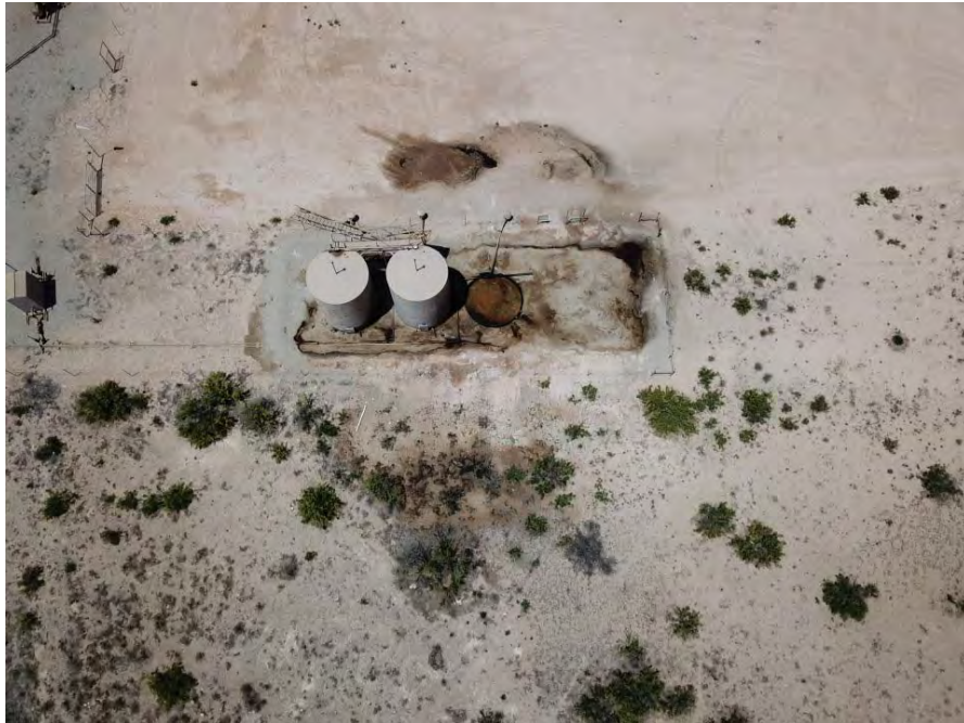
View of site following lightning strike on northern-most tank within the tank battery (Note: This is a drone image with view towards the west)
