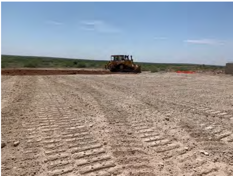
Another view of the site subsequent to the backfill activities.
