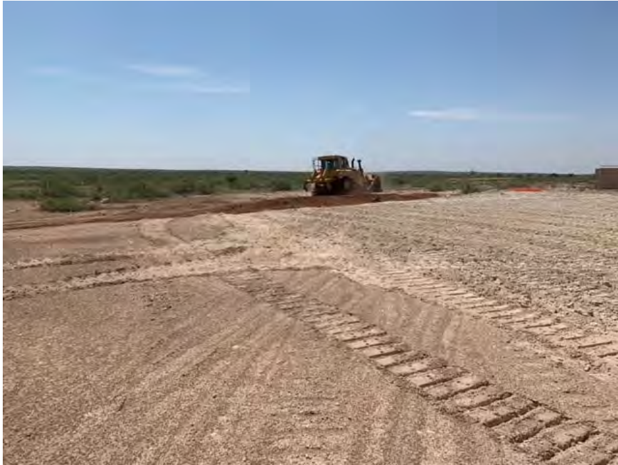
Typical view of the site subsequent to the backfill activities.
