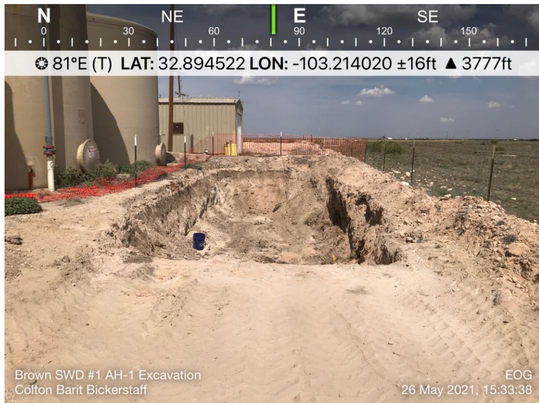
View of Remediation Activities – View Northeast
