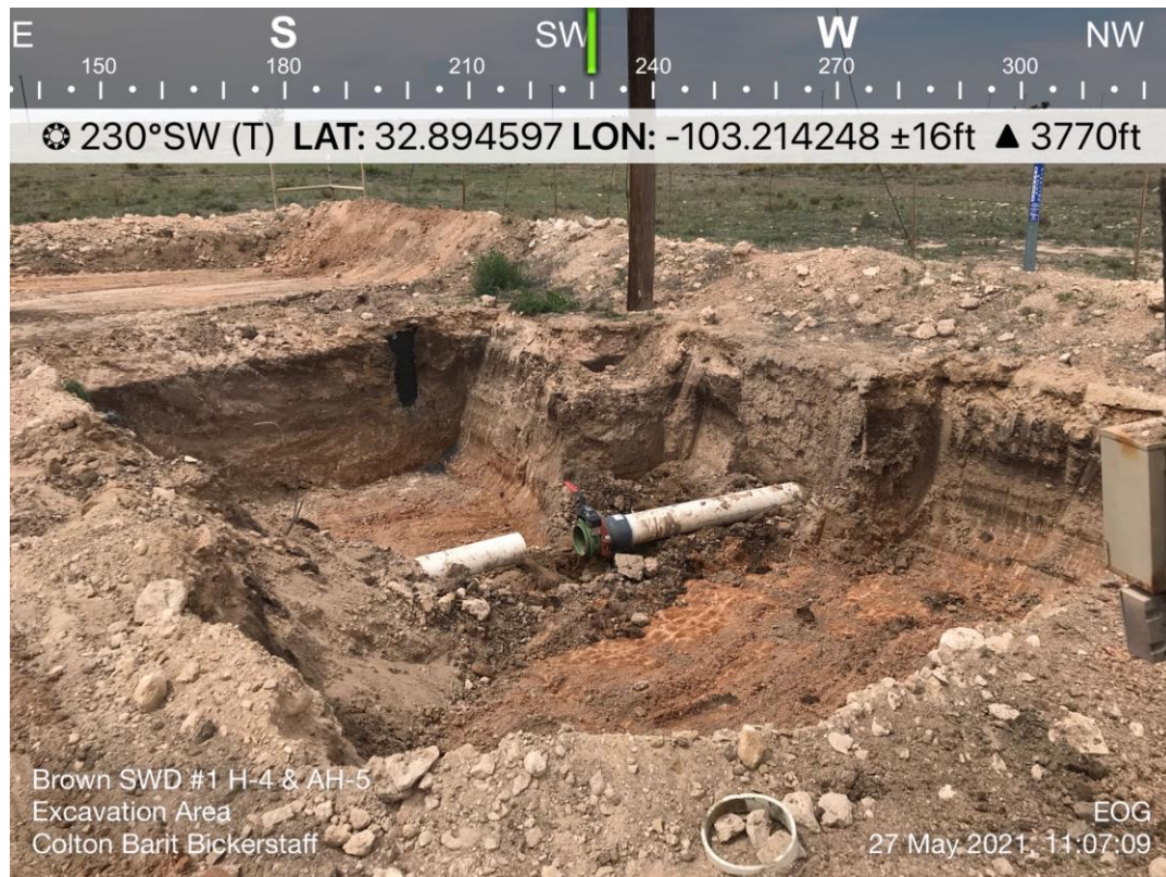
View of Remediation Activities – View Southwest
