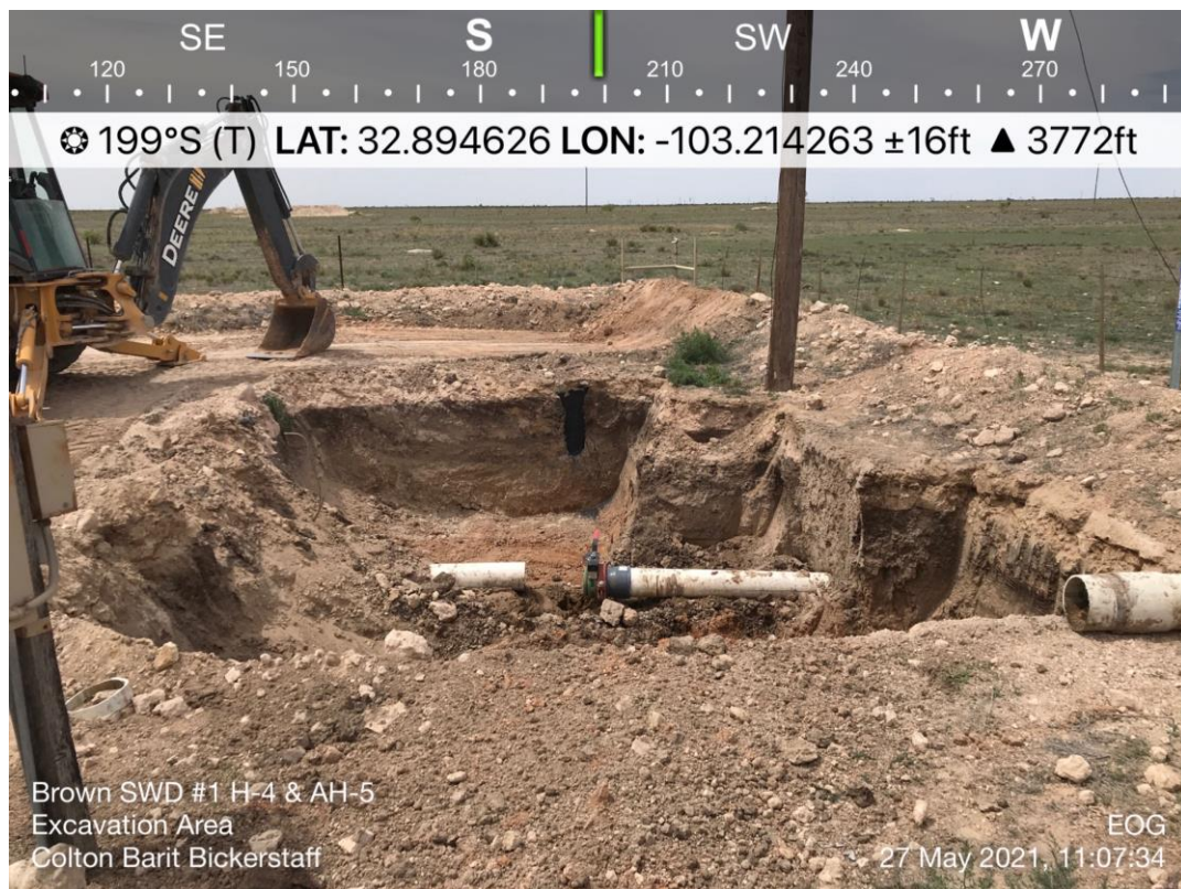
View of Remediation Activities – View South
