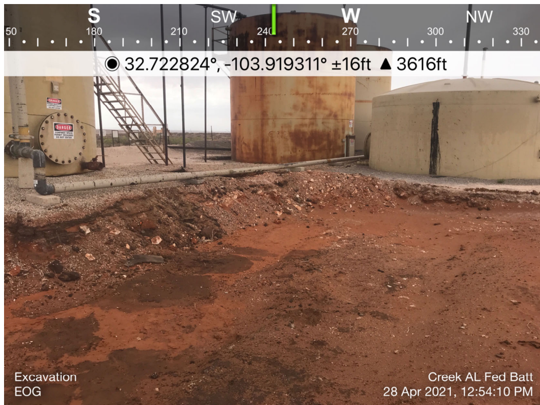
View of Remediation Activities – View Northeast
