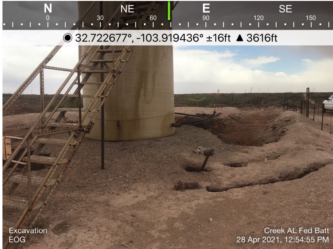
View of Remediation Activities – View Northeast
