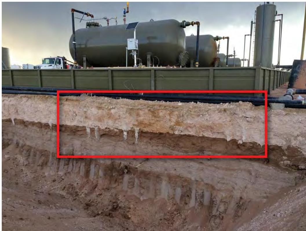
**Photo 4: The red box outlines G-14 Containment Wall (north wall) that is located immediately underneath the tank battery's southern containment wall. Excavation depth is 4.5 feet. TPH exceeds Table 1 Closure Criteria from 0 to 2 feet. The caliche pad is approximately 1-foot thick. G-13 is to the left (west) of G-14 (red outline). Date/Time: 2019-06-25 18:31:01. GPS: 32.4411722 N , -103.5385194 W.**
