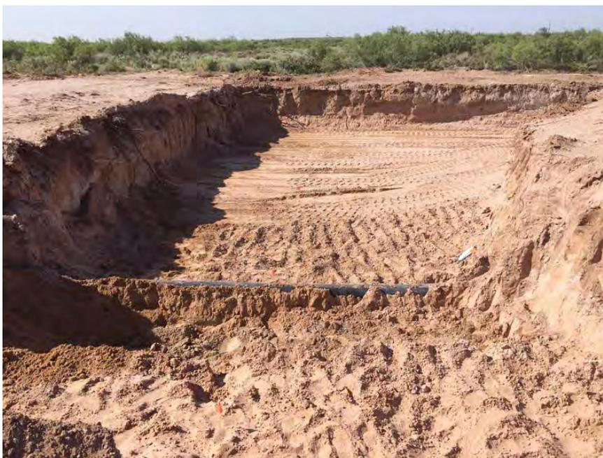
**Photo 5: Excavation from G-01 viewing south toward G-04. A pipeline (G-02) is visible foreground center. Excavation depth from north to south is 4.5, 6.5, 7.5 and 5 feet below ground surface. Date/Time: 2019-06-19 09:06:56. GPS: 32.4412639 N , -103.5382778 W**
