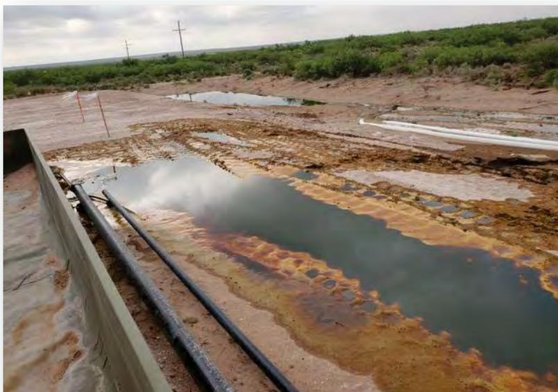
**Photo 1: Crude oil release viewing from the southern edge of the tank battery containment. Photograph is viewing east-southeast. Date: May 25, 2019**
