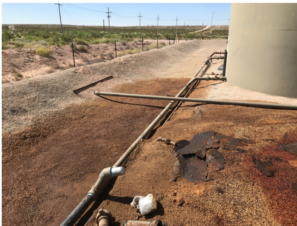
View South – Area of AH-3
