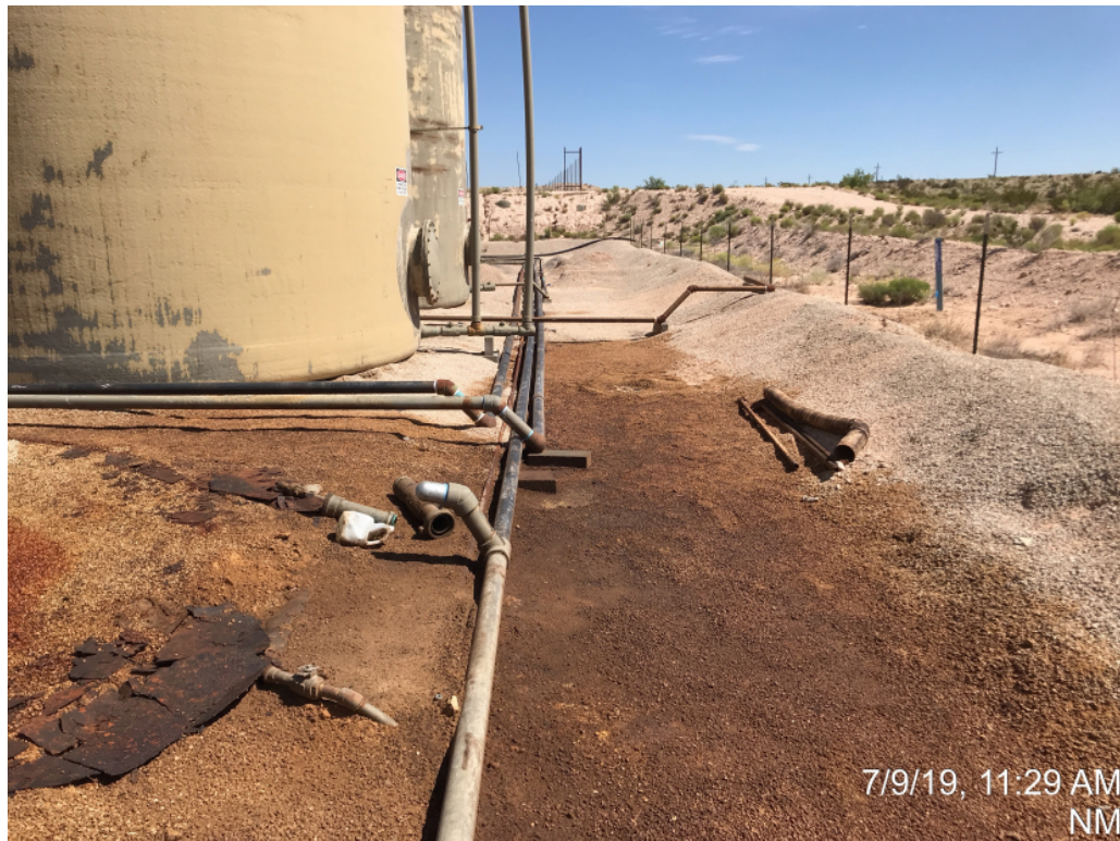
View North – Area of AH-1
