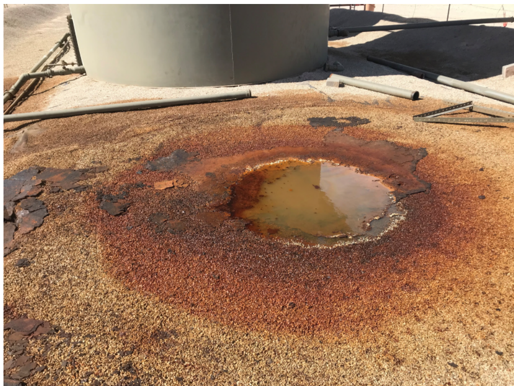
View South – Area of AH-2
