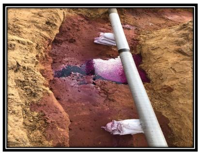
Picture 6: View of Potassium Permanganate Application (View 1)
