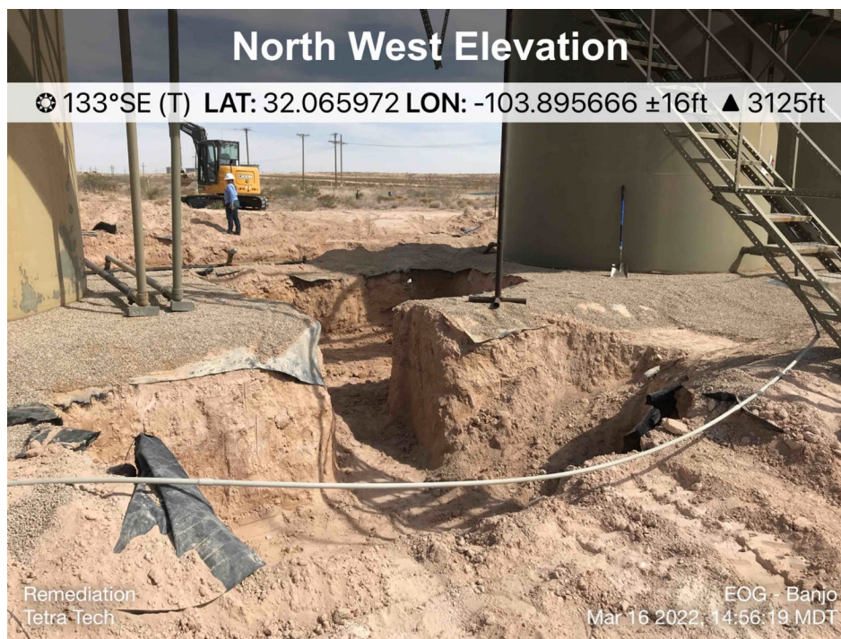
View of Remediation Activities – View Southeast
