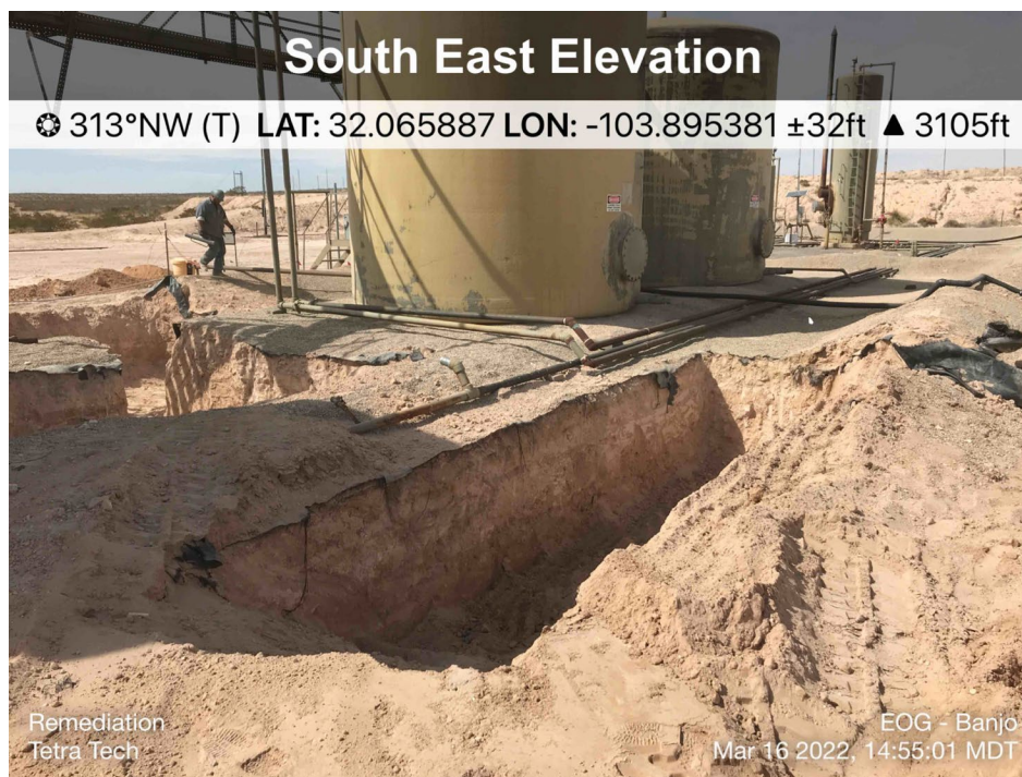
View of Remediation Activities – View Northwest
