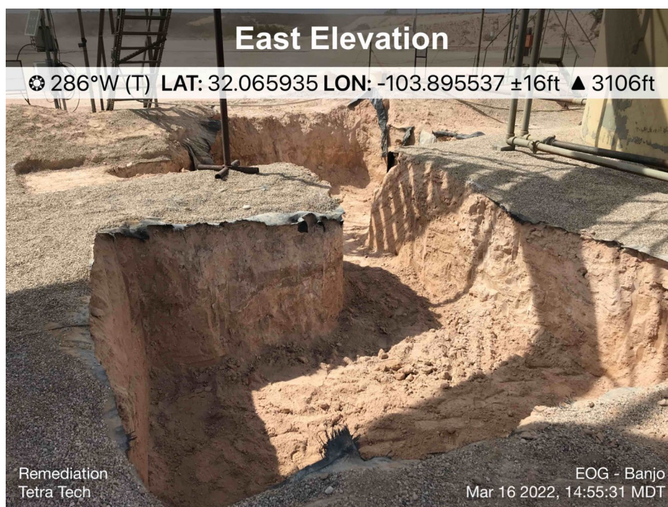
View of Remediation Activities – View West
