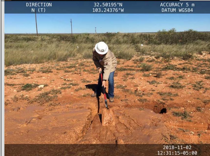
In addition to the standard one-call notification, a hydro-vac was utilized to clear the location prior to sampling due to safety concerns including the presence of flowlines and underground piping. The site is also located near electrical power lines.
