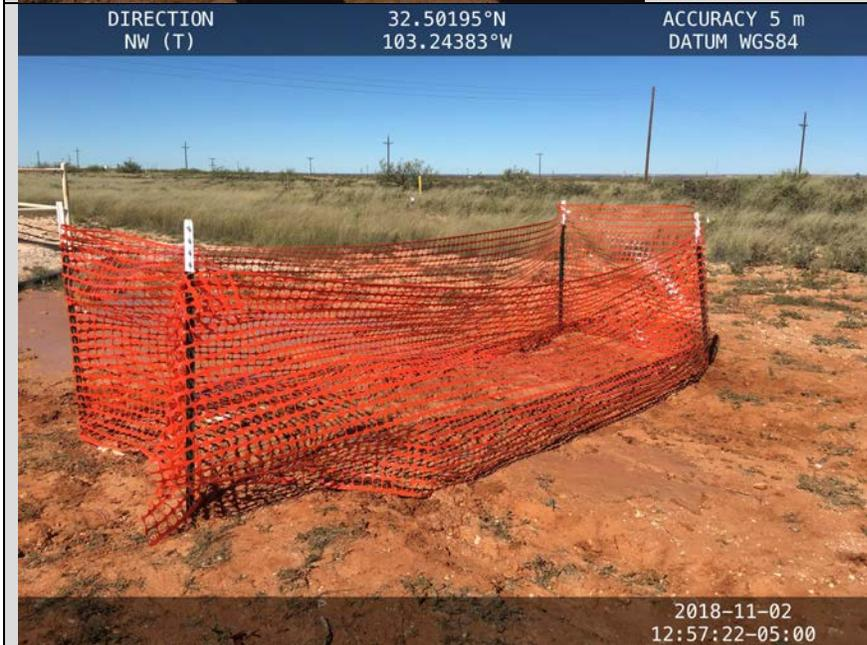
After confirmation soil sampling was complete, the areas that were hydro-vac'ed were enclosed with orange mesh safety fencing as a protective measure.
