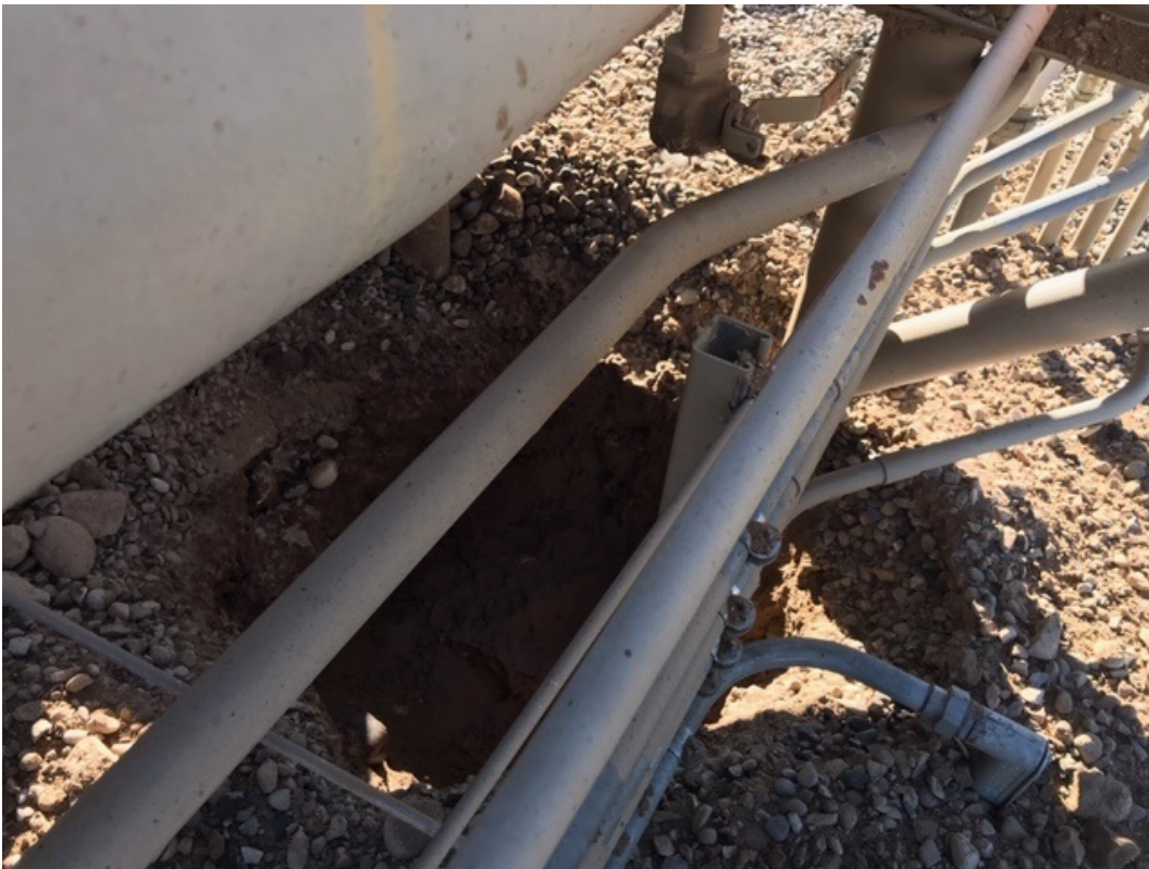
Photo 2: Hole created by released gas.
