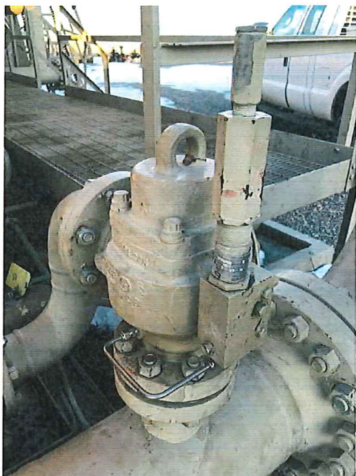
Photo 1: Safety relief valve with new pneumatic supply line.
