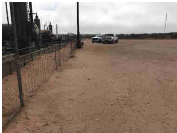
Photograph 7: View of release area (2RP-3440 & 2RP-4914), facing south.
