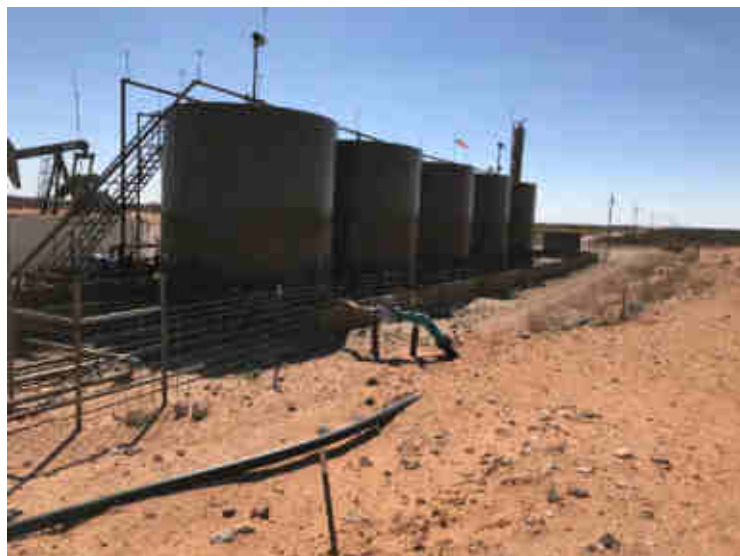
Photograph 3: View of release area (2RP-3985), facing west.
