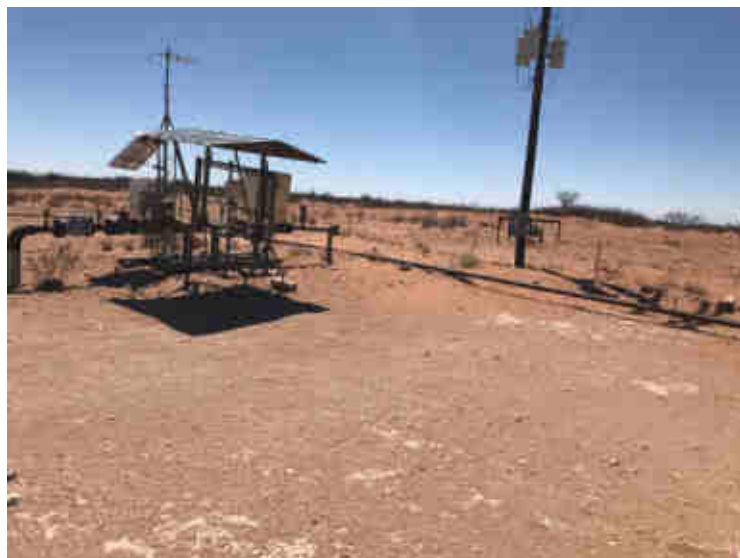
Photograph 1: View of release area (2RP-3440), facing southwest.
