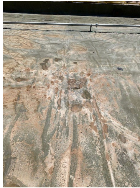
Photograph 4 Date: June 7, 2022 Description: Patched liner following delineation activities
