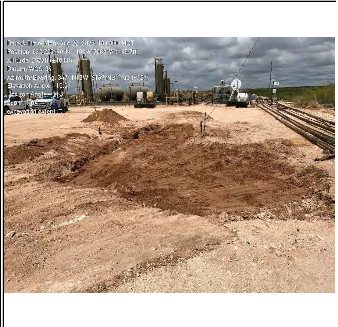
Photograph 4 Date: August 22, 2022 Description: View of final excavation extent, facing northwest.
