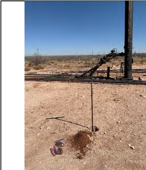
Photograph 3 Date: February 14, 2021 Description: View of delineation activities, facing east.
