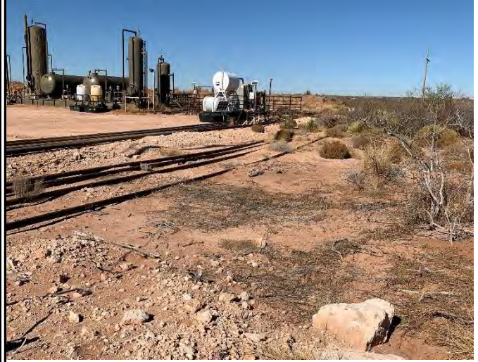
Photograph 2 Date: November 29, 2021 Description: View of flare area, facing northwest.
