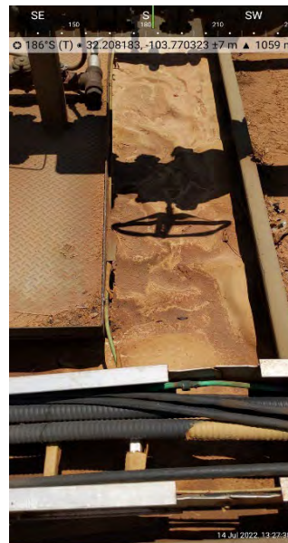
Photograph 2 Date: July 13, 2022 Description: View of liner during containment inspection facing south.
