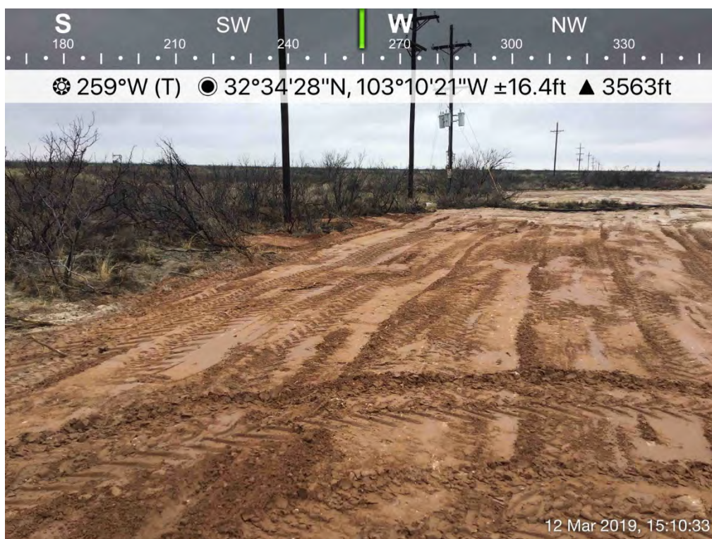
Backfilled Excavation (SP-15/Historical Release)
