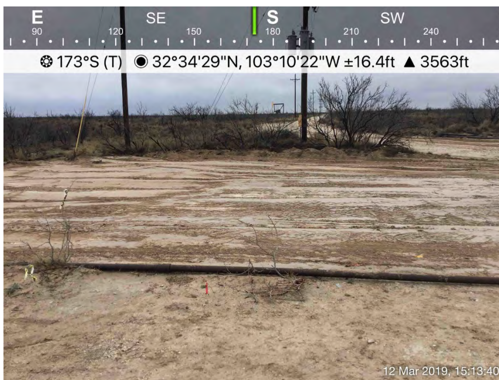
Backfilled Excavation (SP-2 &amp; SP-4, in background)
