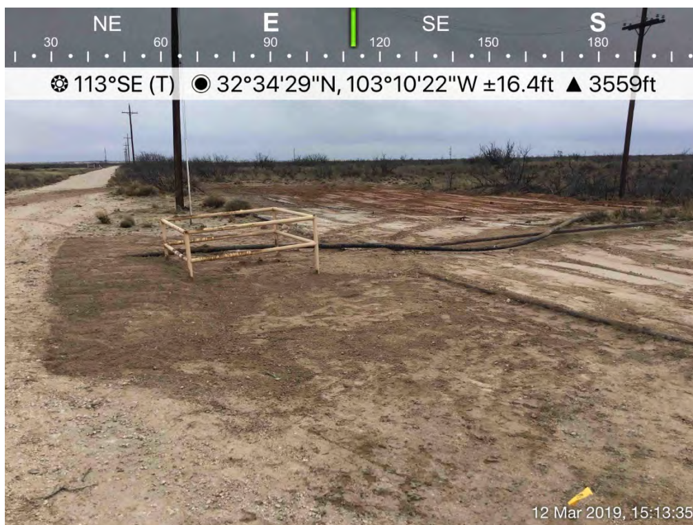
Backfilled Excavation (SP-2 &amp; SP-15/Historical Release, in background)
