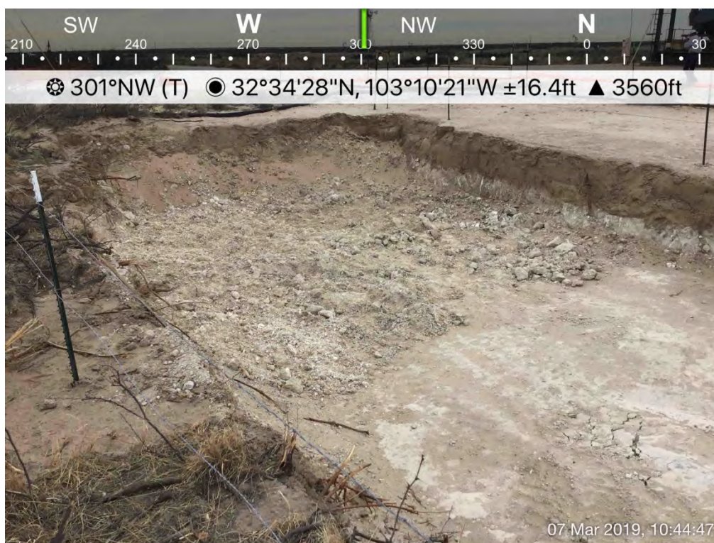
Excavation (SP-15/Historical Release)
