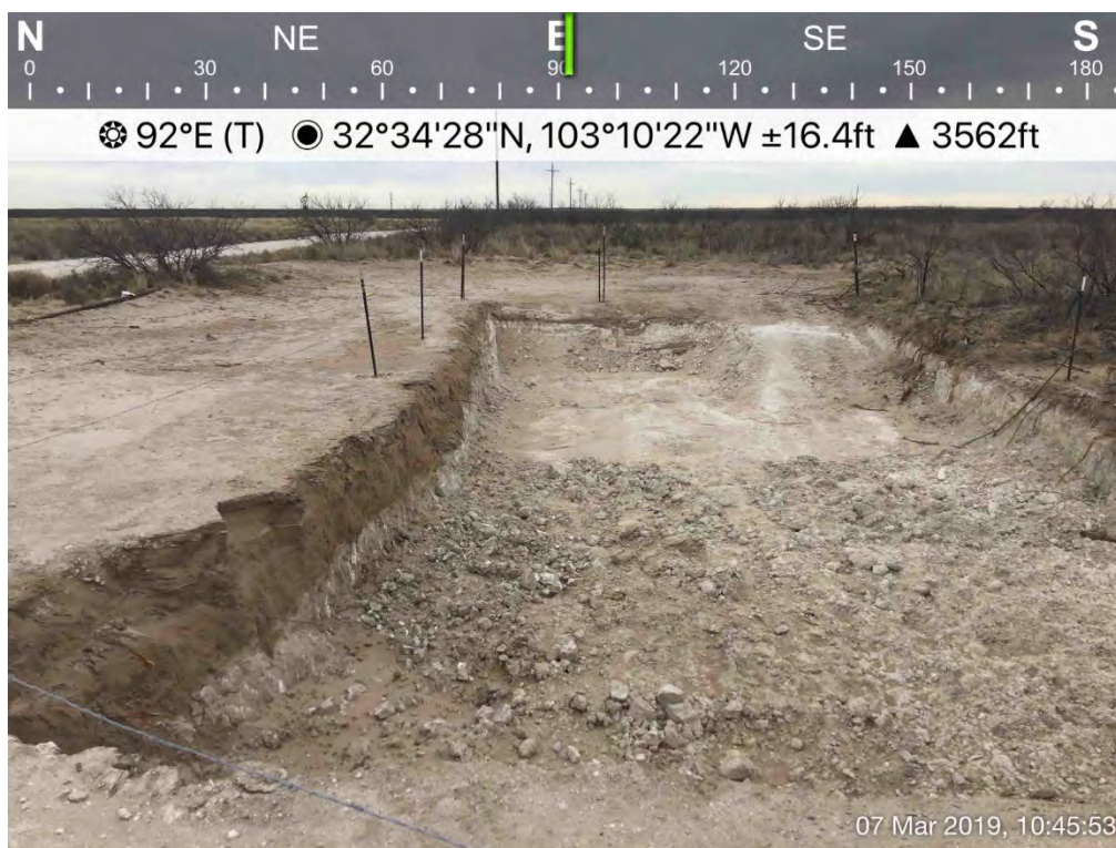
Excavation (SP-15/Historical Release)
