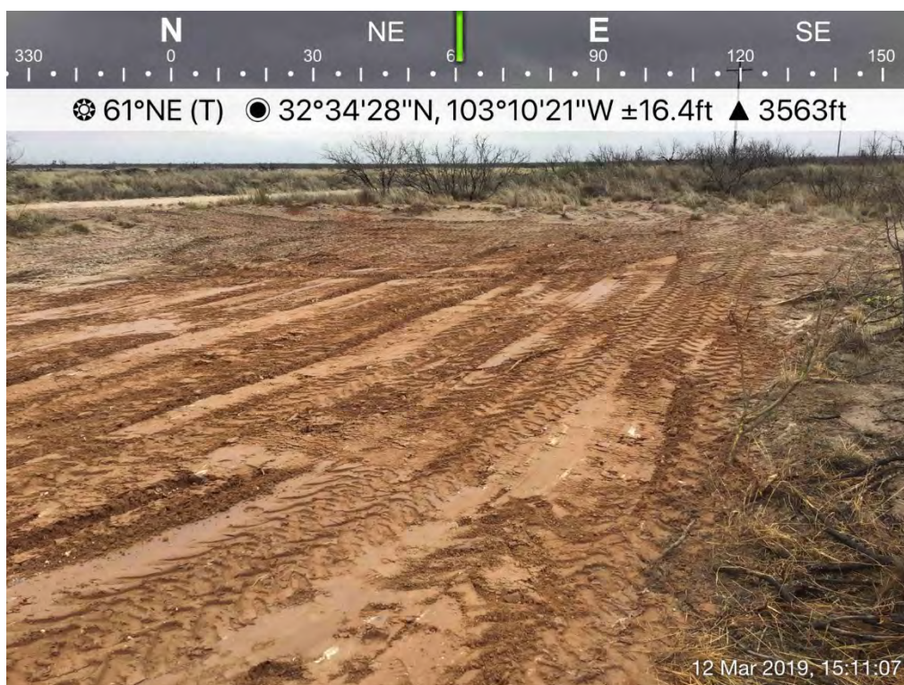
Backfilled Excavation (SP-15/Historical Release)
