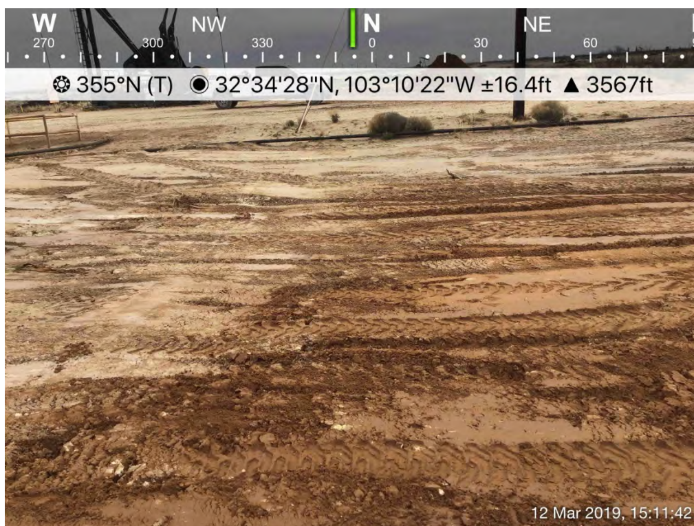
Backfilled Excavation (SP-15/Historical Release)
