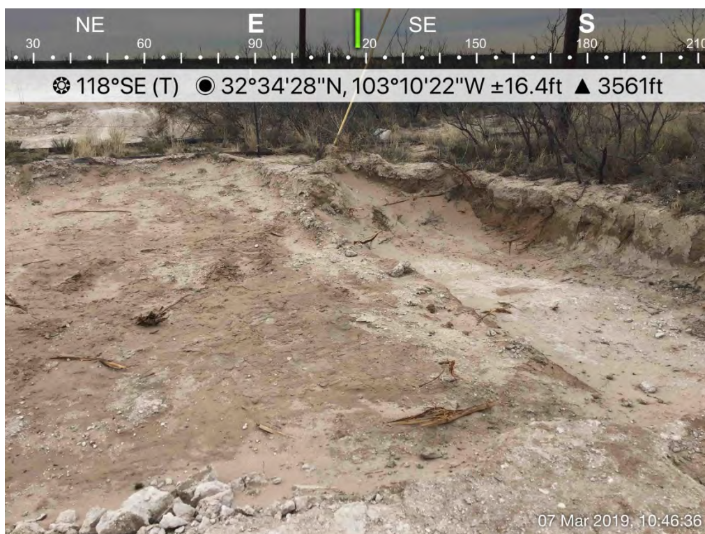
Excavation (SP-2 &amp; SP-4)
