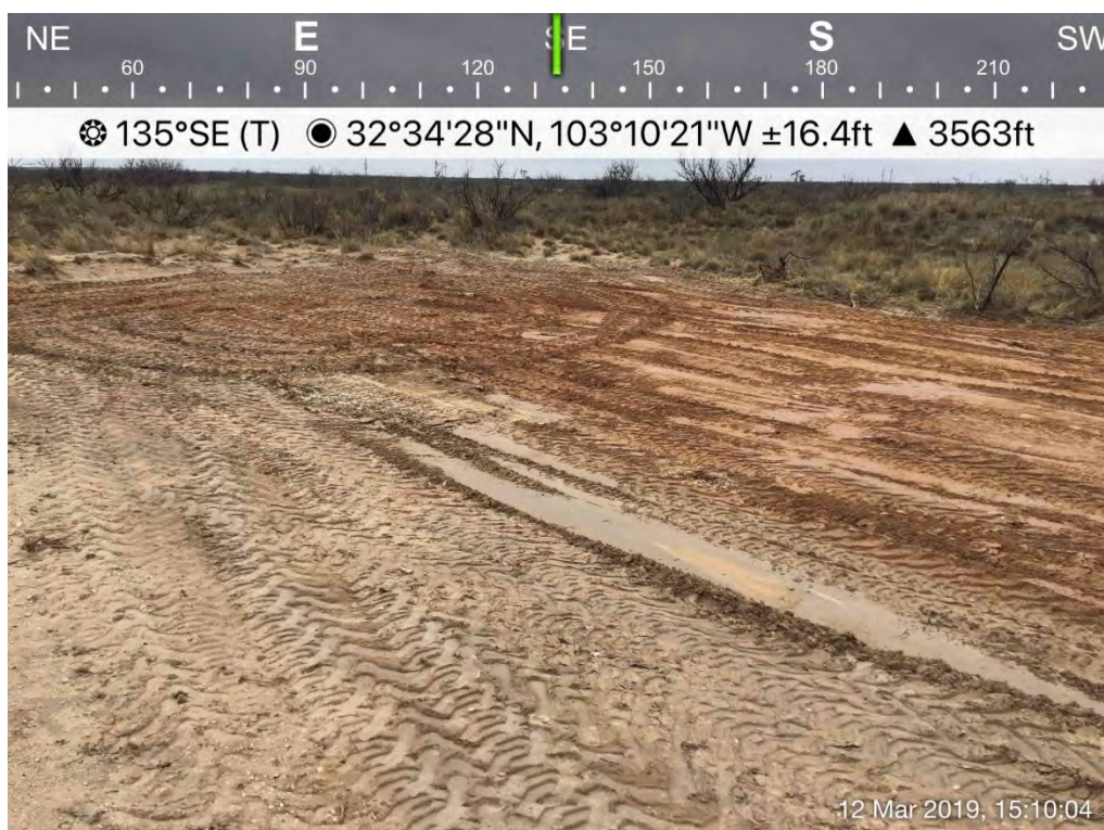
Backfilled Excavation (SP-15/Historical Release)
