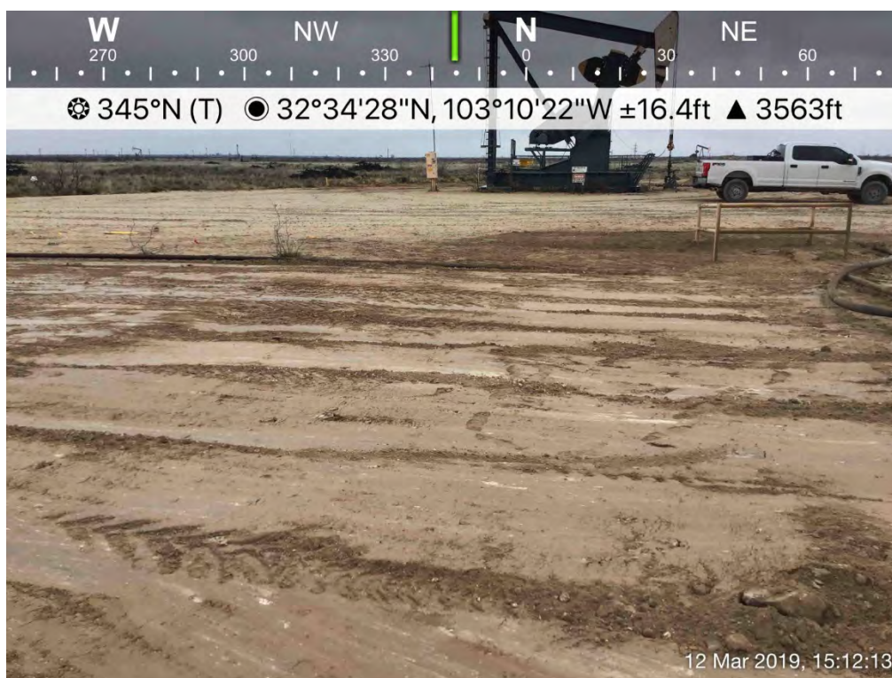
Backfilled Excavation (SP-2)
