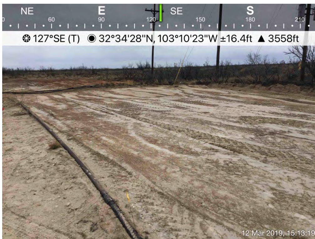
Backfilled Excavation (SP-2)
