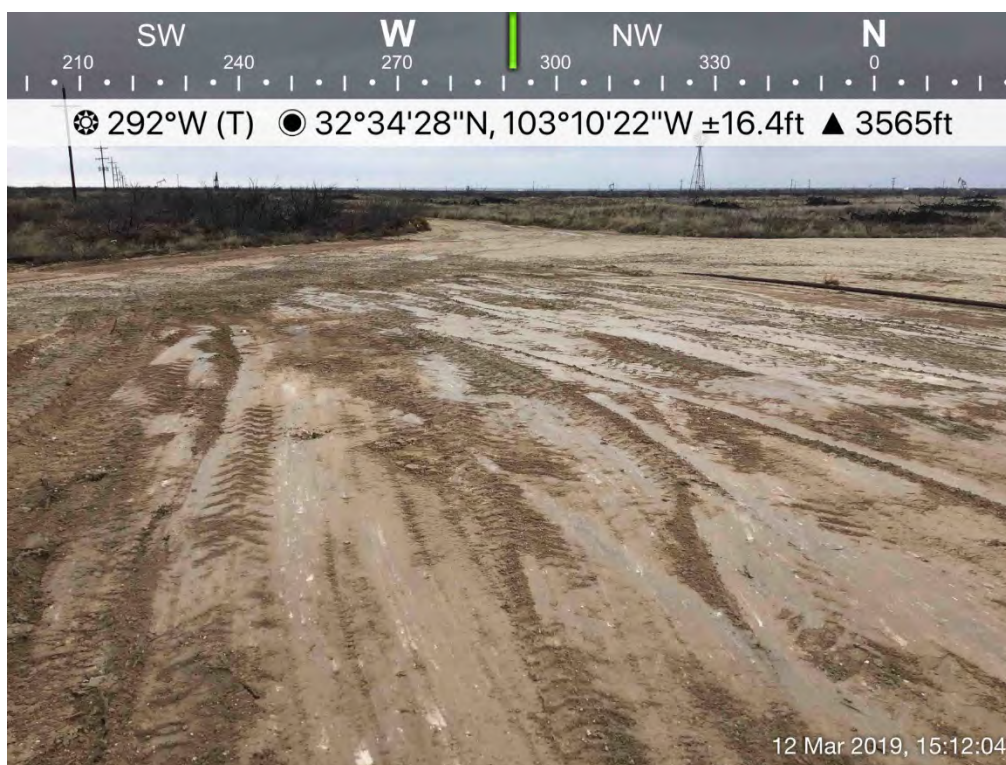
Backfilled Excavation (SP-2 &amp; SP-6, in background)
