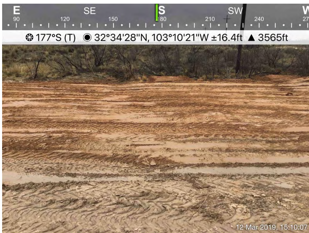
Backfilled Excavation (SP-15/Historical Release)
