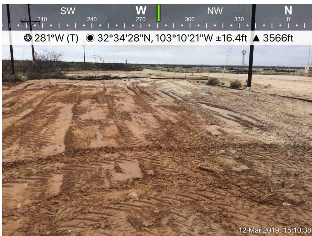
Backfilled Excavation (SP-15/Historical Release)
