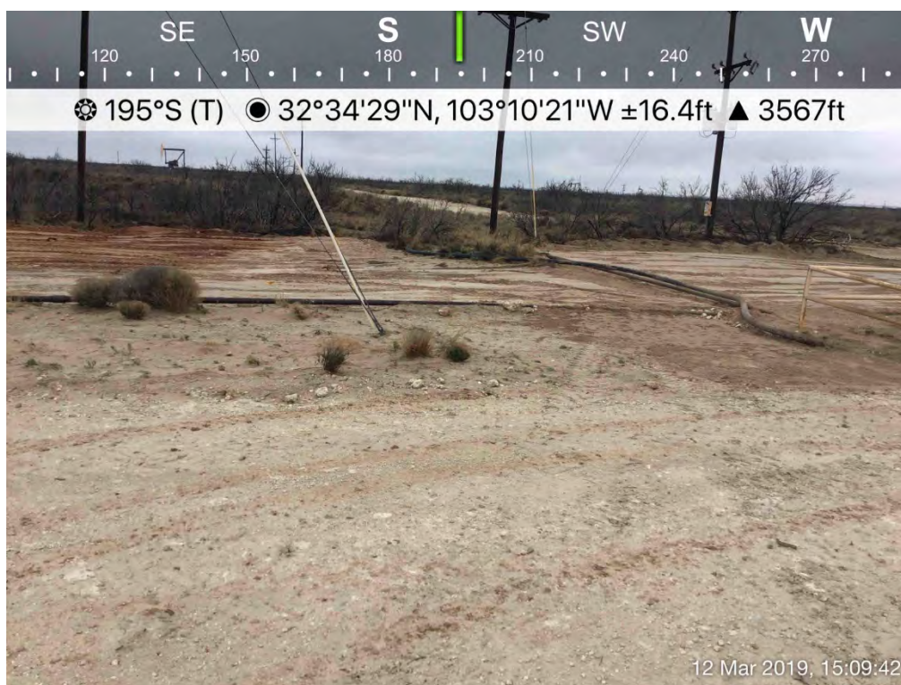
Backfilled Excavation (SP-15/Historical Release &amp; SP-2, in right background)
