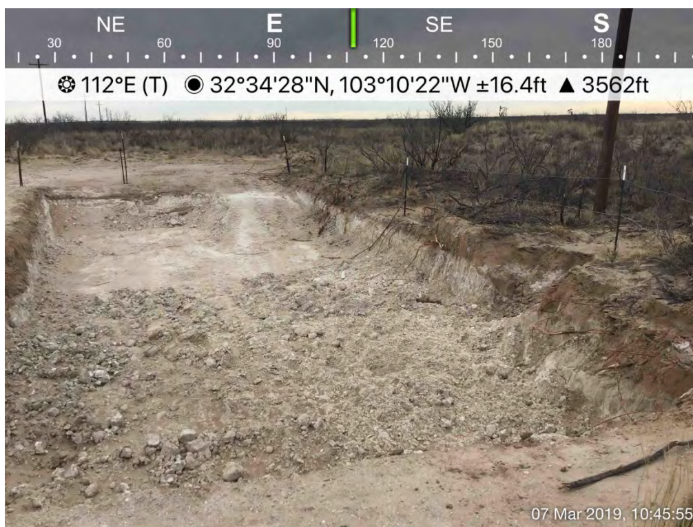
Excavation (SP-15/Historical Release)
