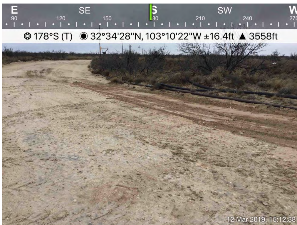
Backfilled Excavation (SP-6)
