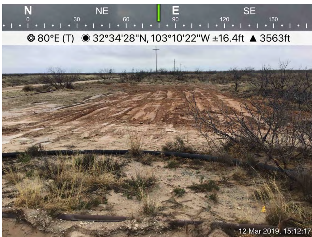
Backfilled Excavation (SP-15/Historical Release)
