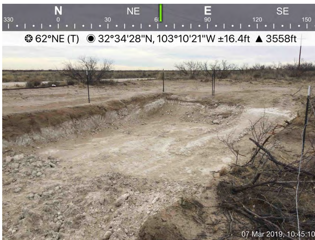
Excavation (SP-15/Historical Release)
