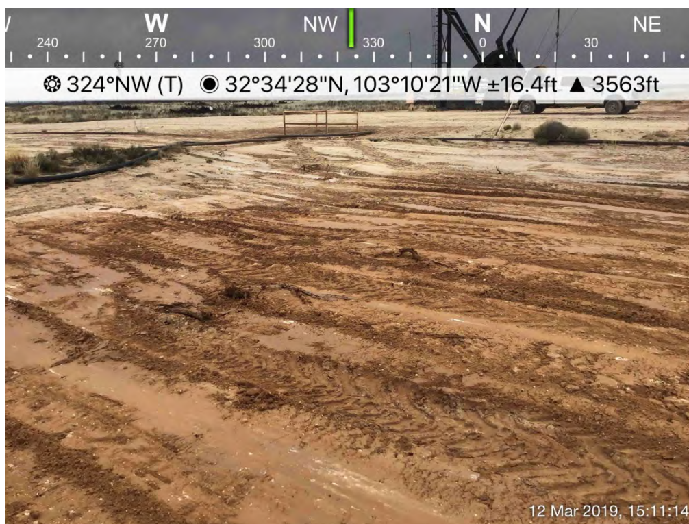
Backfilled Excavation (SP-15/Historical Release)
