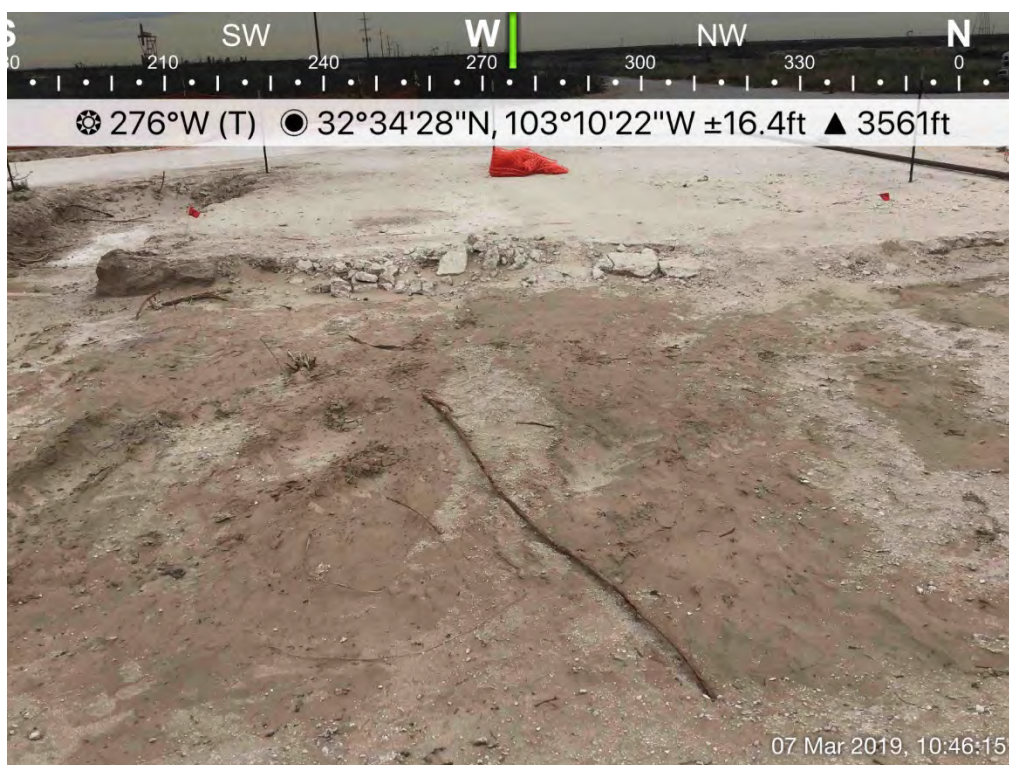
Excavation (SP-2 &amp; SP-4, in left background)
