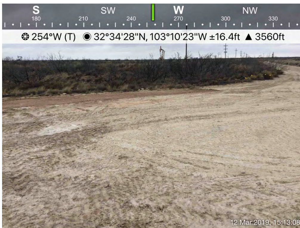
Backfilled Excavation (SP-6)
