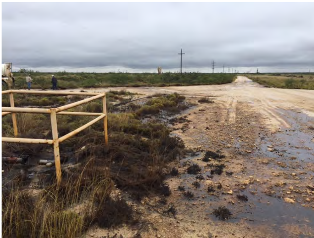
Release (Looking West-Southwest)
