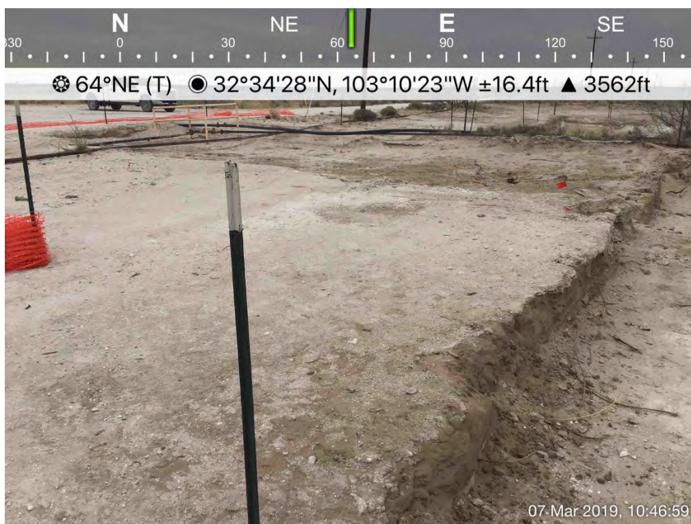
Excavation (SP-2 &amp; SP-4)
