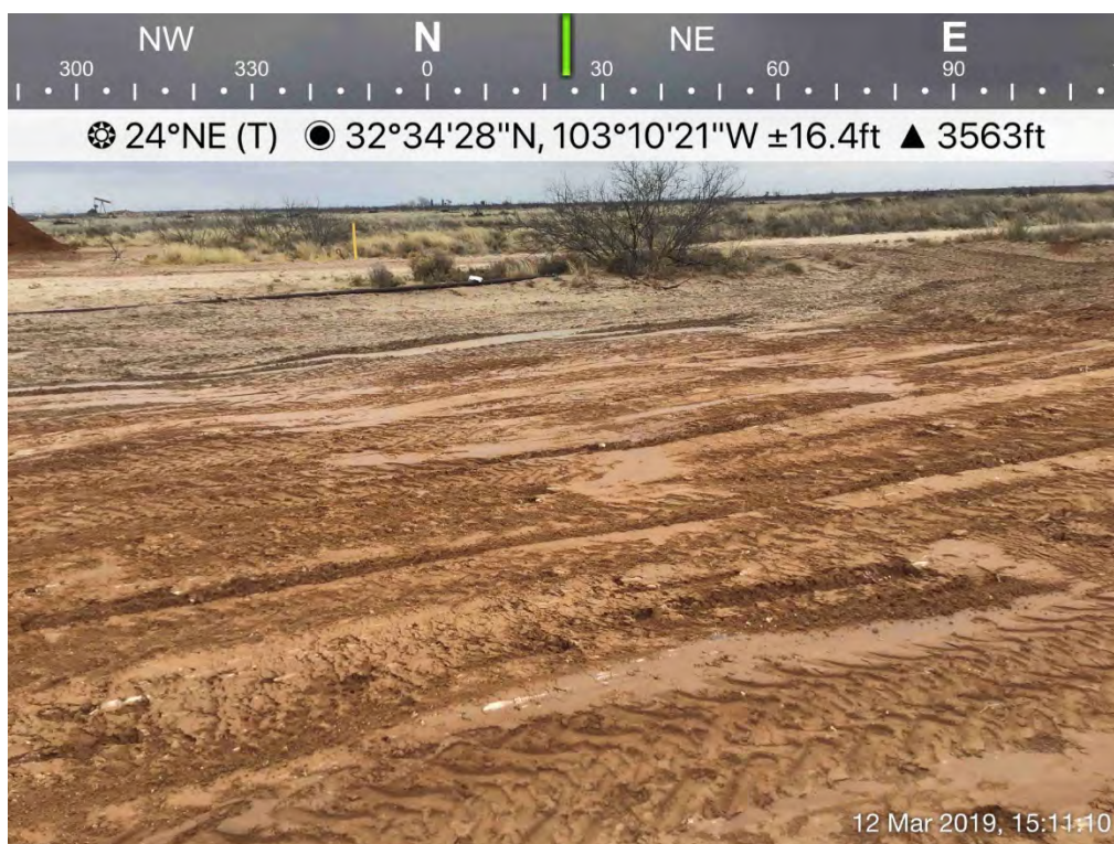
Backfilled Excavation (SP-15/Historical Release)
