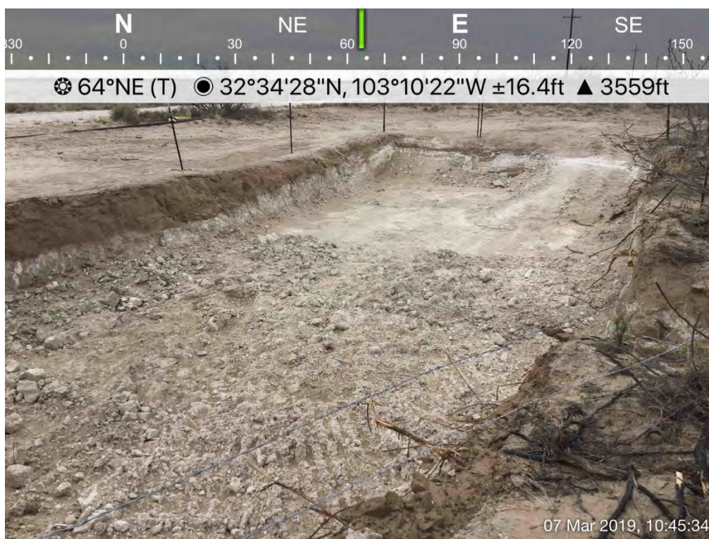
Excavation (SP-15/Historical Release)
