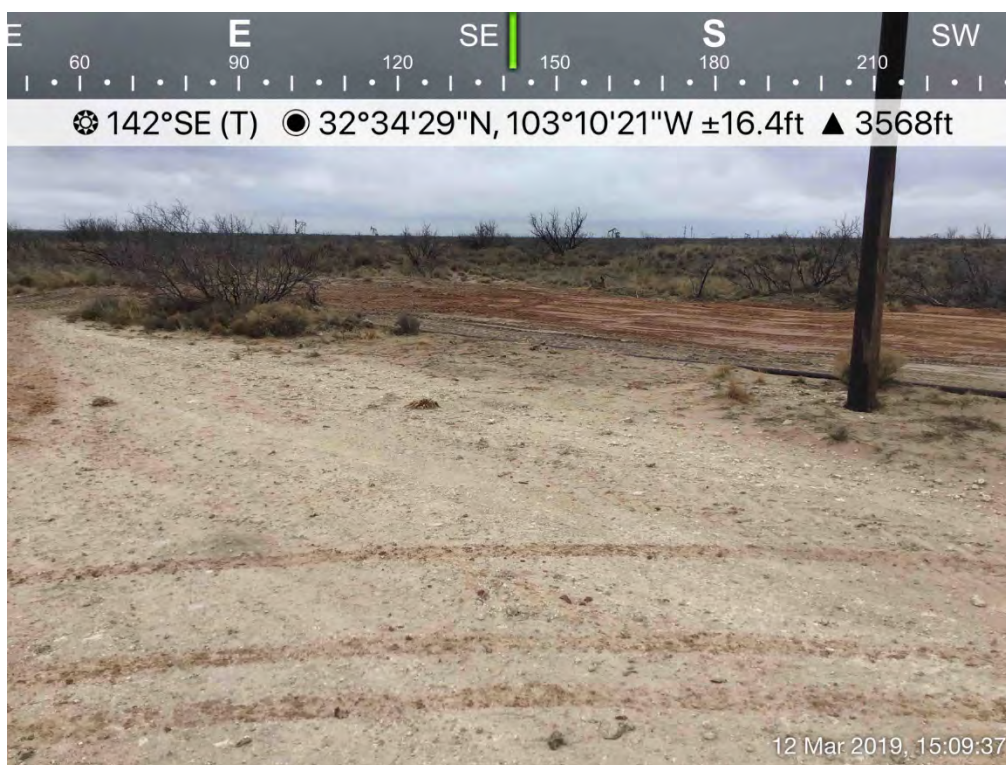
Backfilled Excavation (SP-15/Historical Release)
