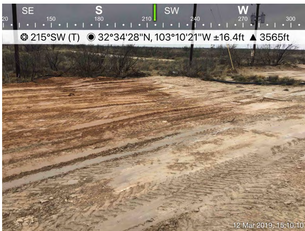
Backfilled Excavation (SP-15/Historical Release)
