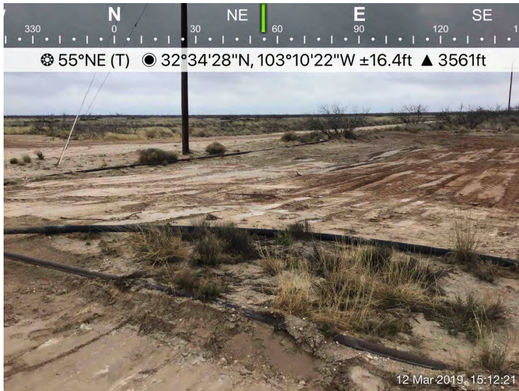
Backfilled Excavation (SP-15/Historical Release)
