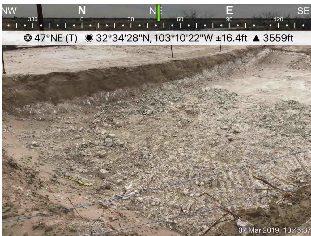
Excavation (SP-15/Historical Release)
