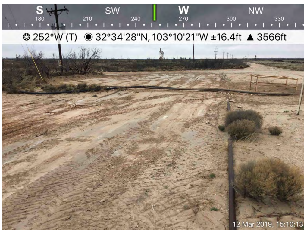
Backfilled Excavation (SP-15/Historical Release &amp; SP-2, in background)
