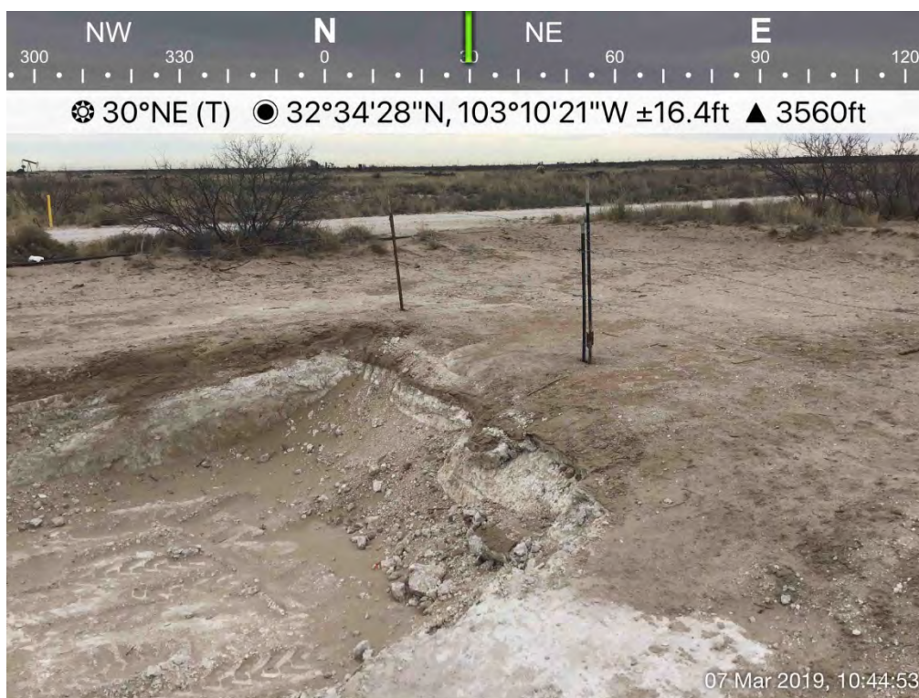
Excavation (SP-15/Historical Release)
