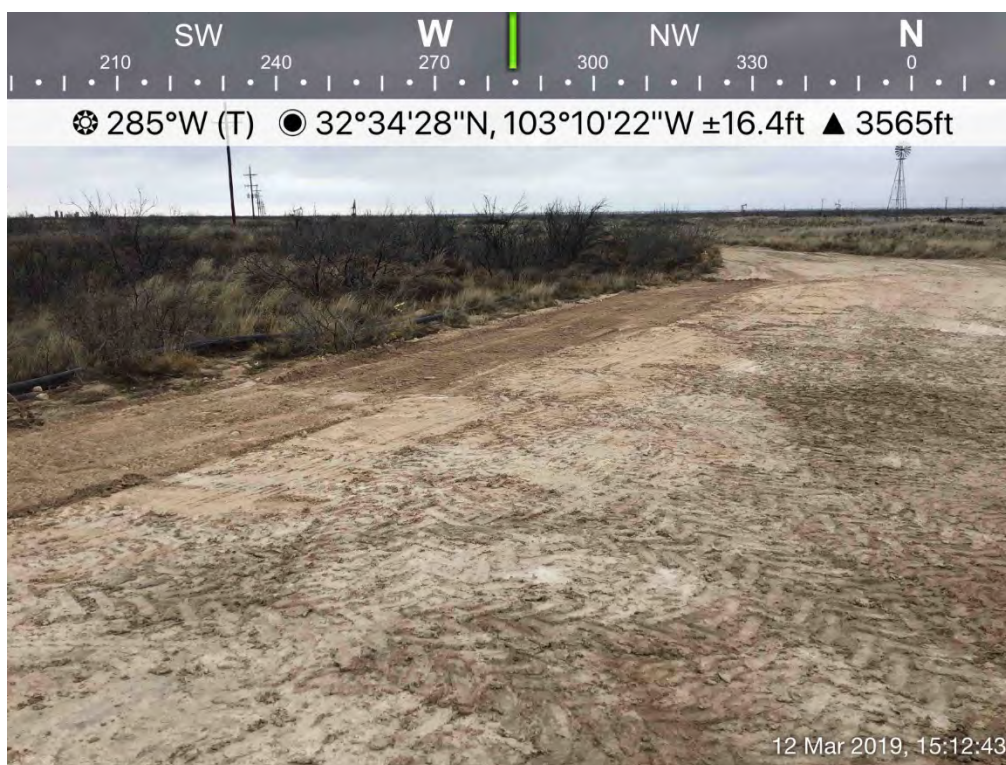
Backfilled Excavation (SP-6)
