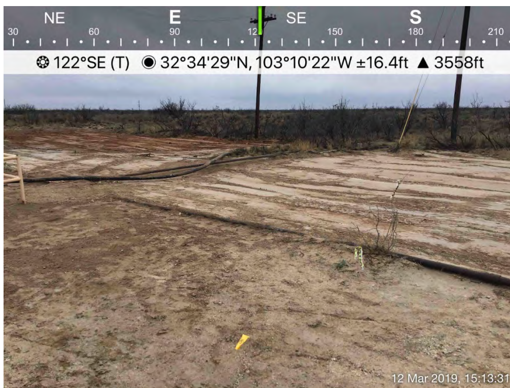
Backfilled Excavation (SP-2 &amp; SP-15/Historical Release, left background)
