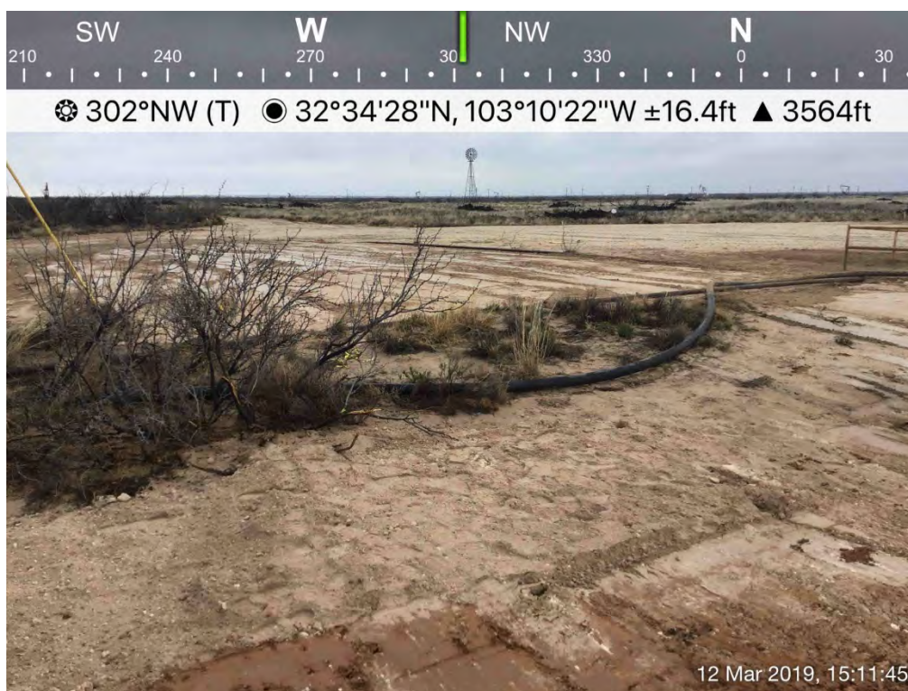
Backfilled Excavation (SP-2, in background &amp; SP-15/Historical Release, in foreground)
