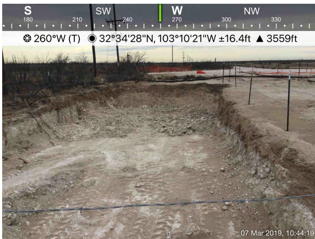
Excavation (SP-15/Historical Release)
