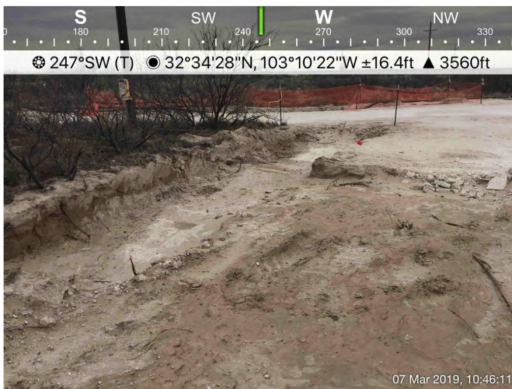
Excavation (SP-2/SP-4, in foreground &amp; SP-6, in background)
