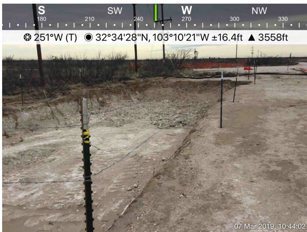
Excavation (SP-15/Historical Release)
