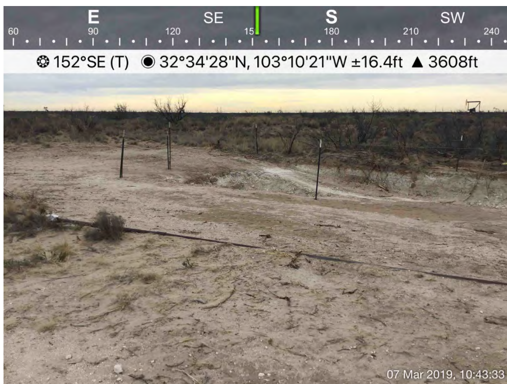
Excavation (SP-15/Historical Release)
