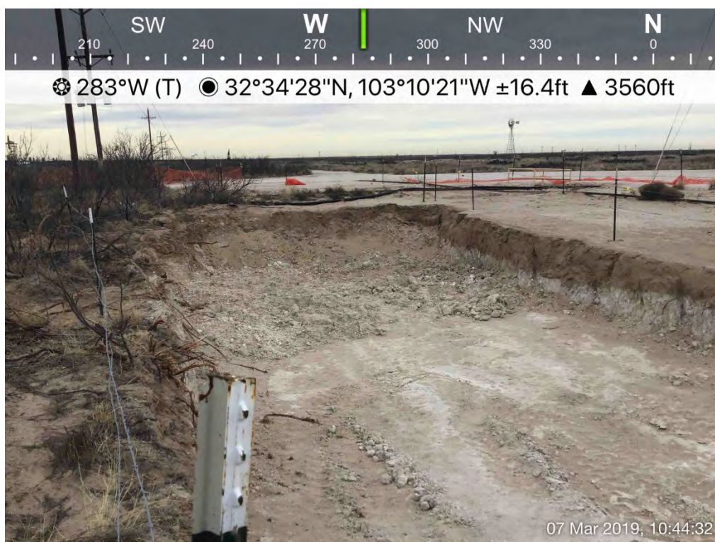
Excavation (SP-15/Historical Release)
