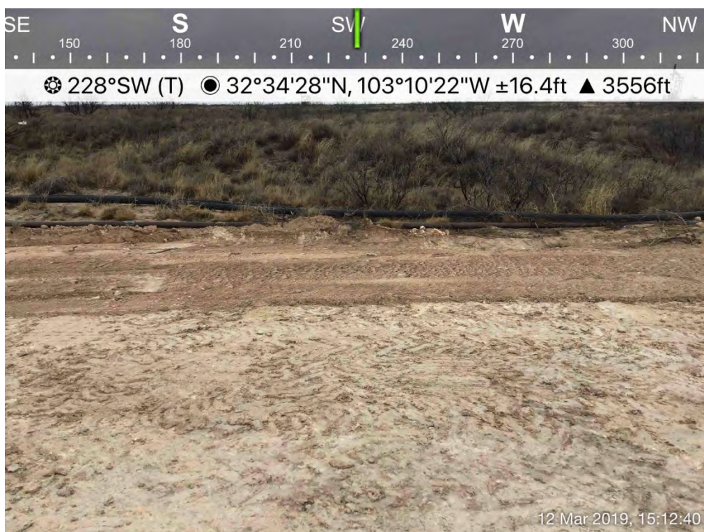
Backfilled Excavation (SP-6)
