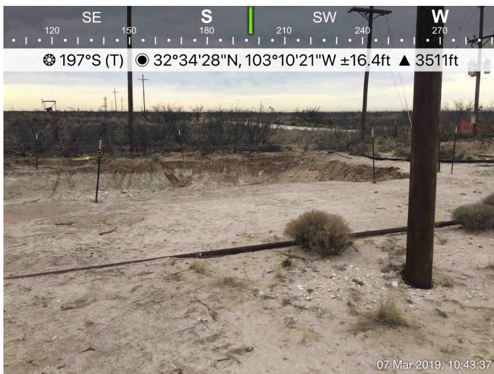
Excavation (SP-15/Historical Release)
