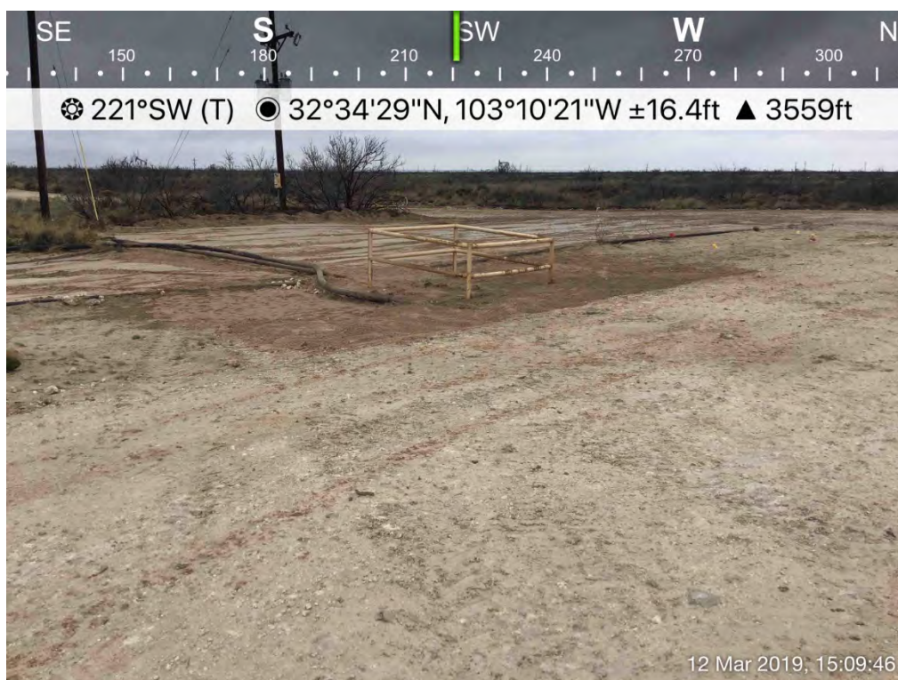
Backfilled Excavation (SP-2)
