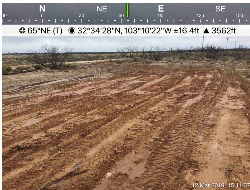
Backfilled Excavation (SP-15/Historical Release)
