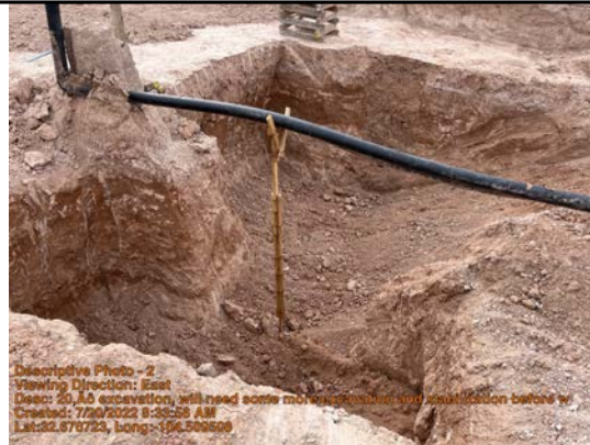
20' excavation, will need some more excavation and stabilization before we can sample
