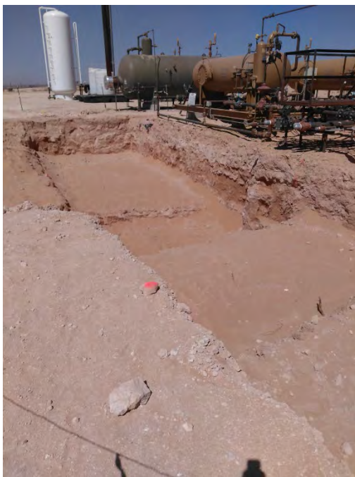
Photo 10: West view of the northwestern corner of the excavation.
