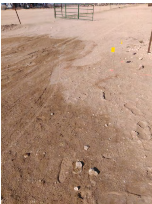
Photo 4: West view of westernmost end of visibly affected area.
