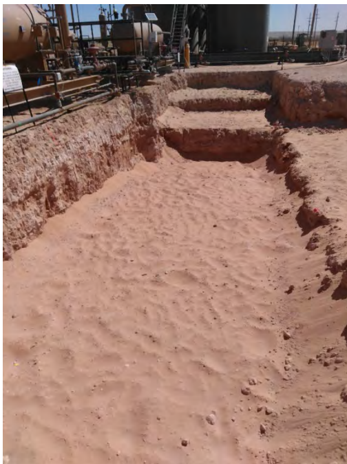
Photo 8: East view of the eastern end of the excavation.
