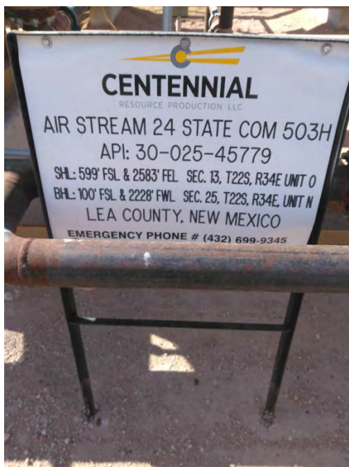
Photo 1: Lease sign at the Airstream 24 State Com 503H-504H Tank Battery.
