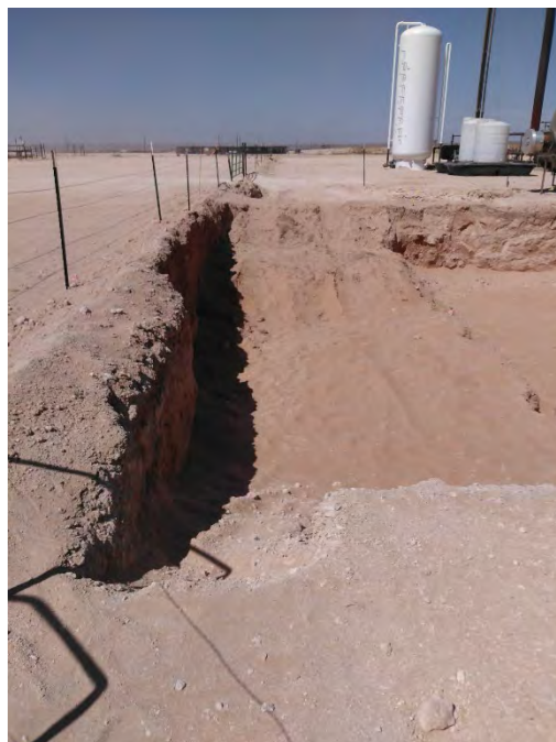
Photo 11: West view of the southwest corner of the excavation.
