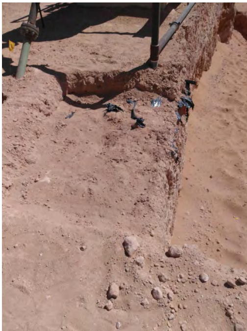
Photo 7: East view of preexisting liner encountered during excavation on March 28, 2022.
