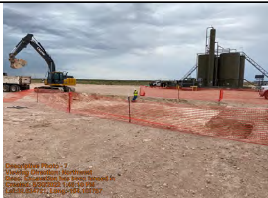
Excavation has been fenced in and will be closed at the end of the day
