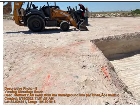
Marked 2' away from the underground line per Chad's instruction
