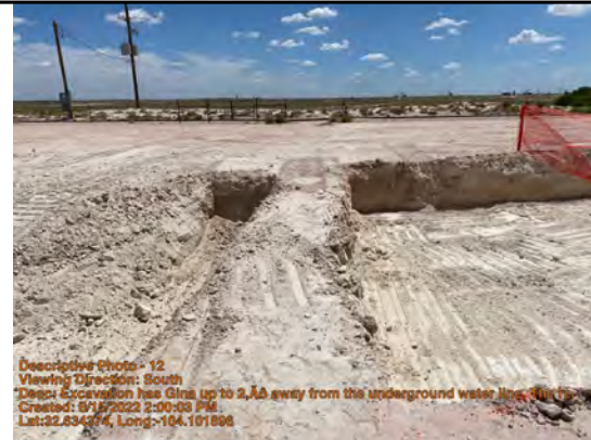
Excavation has Gina up to 2' away from the underground water line. The rest will be done by hand
