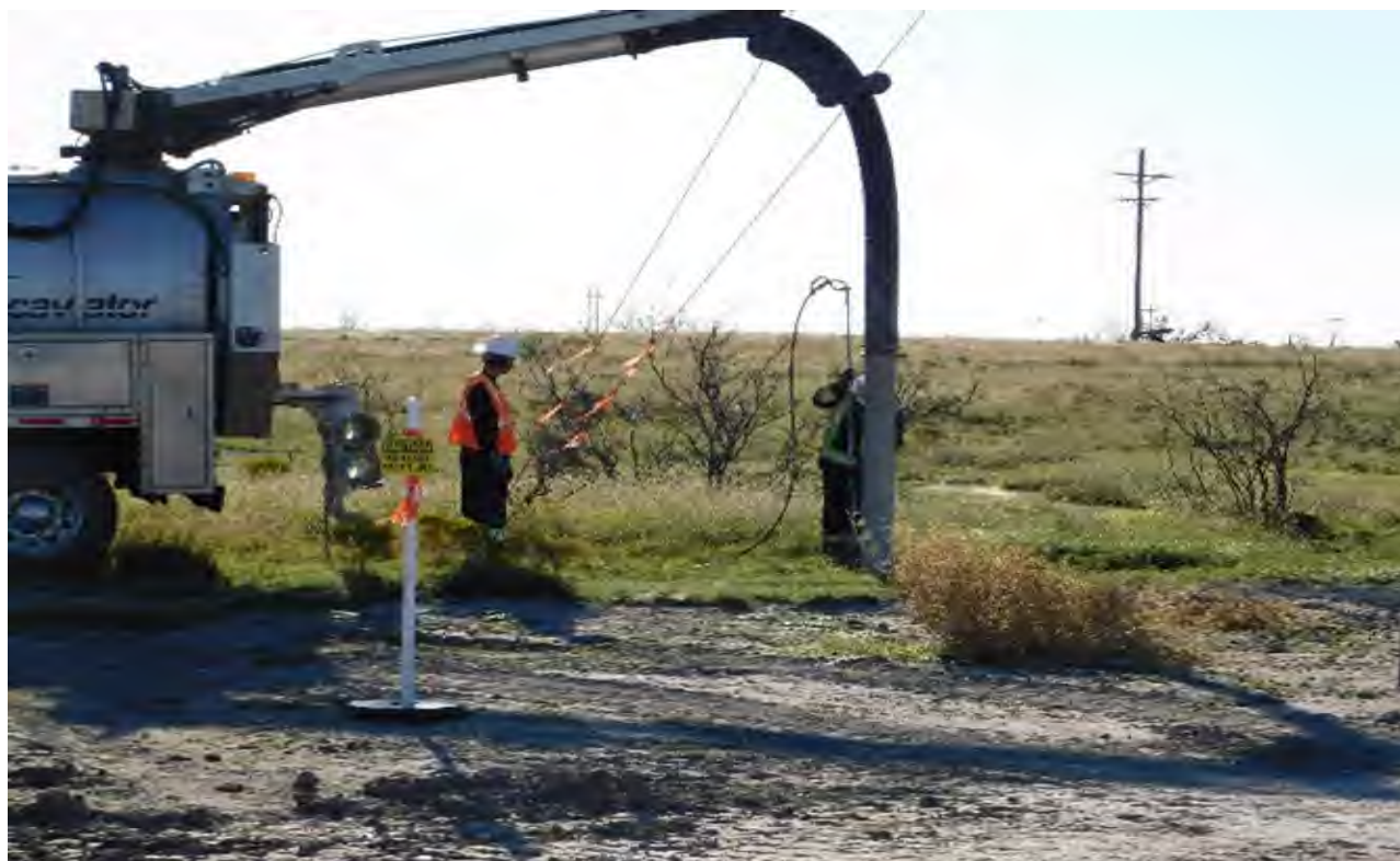
Photo 1. View of hydro excavation activities.
