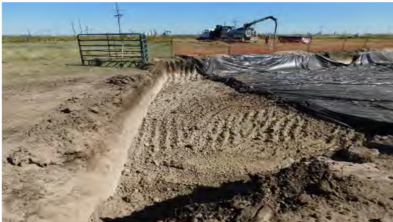
Photo 5. View of liner installation.
