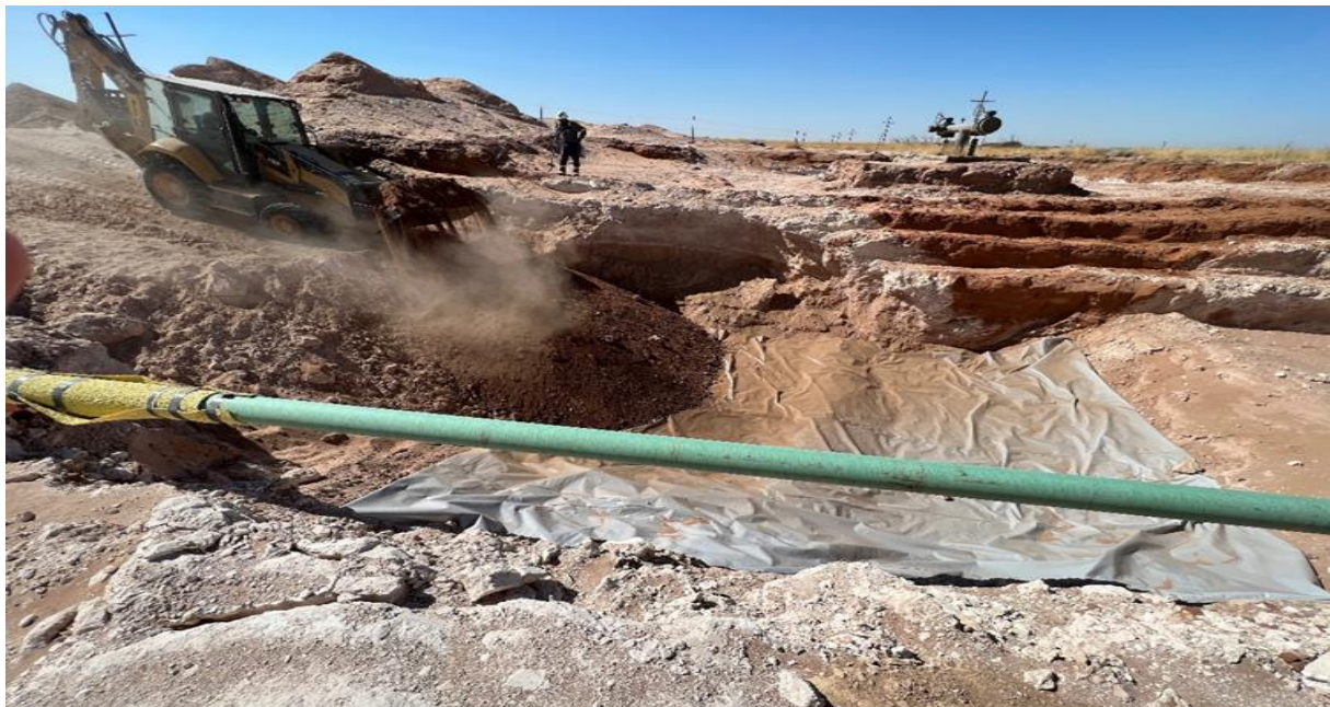
Photo 6 Liner installation and backfill activities.
