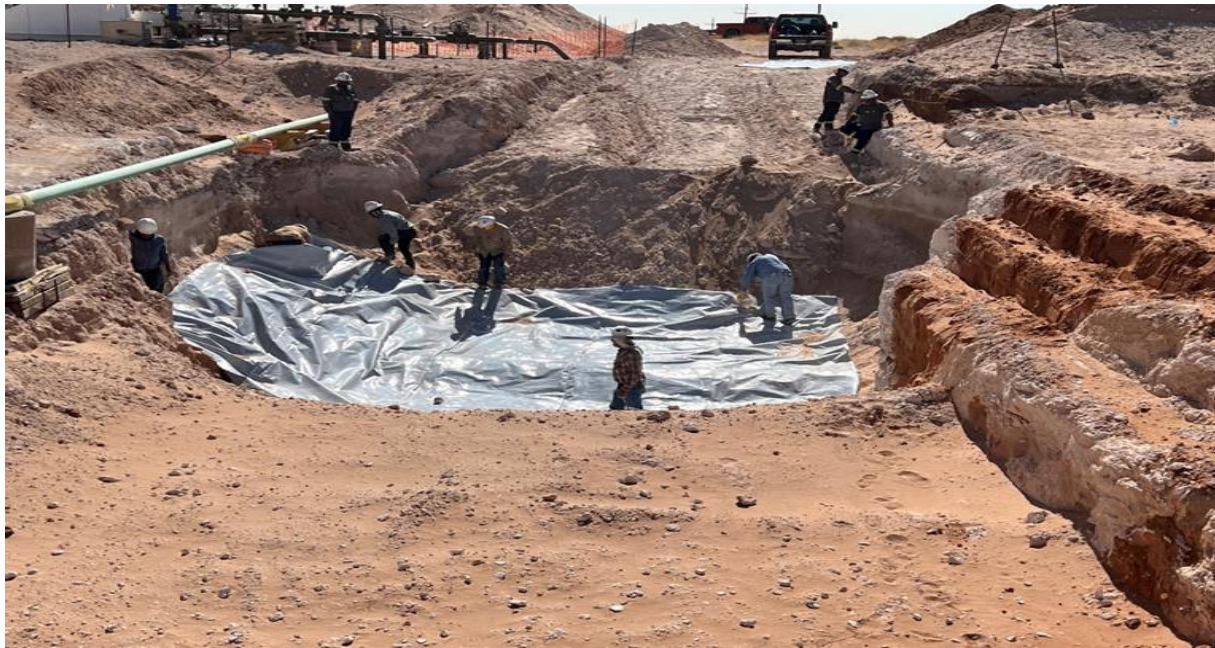
Photo 5 Liner installation during backfill activities.
