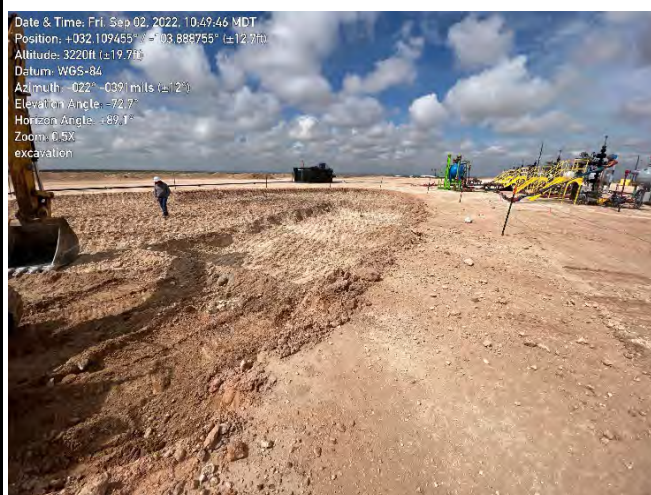
Photograph 4 Date: September 2, 2022 Description: Excavation Activities
