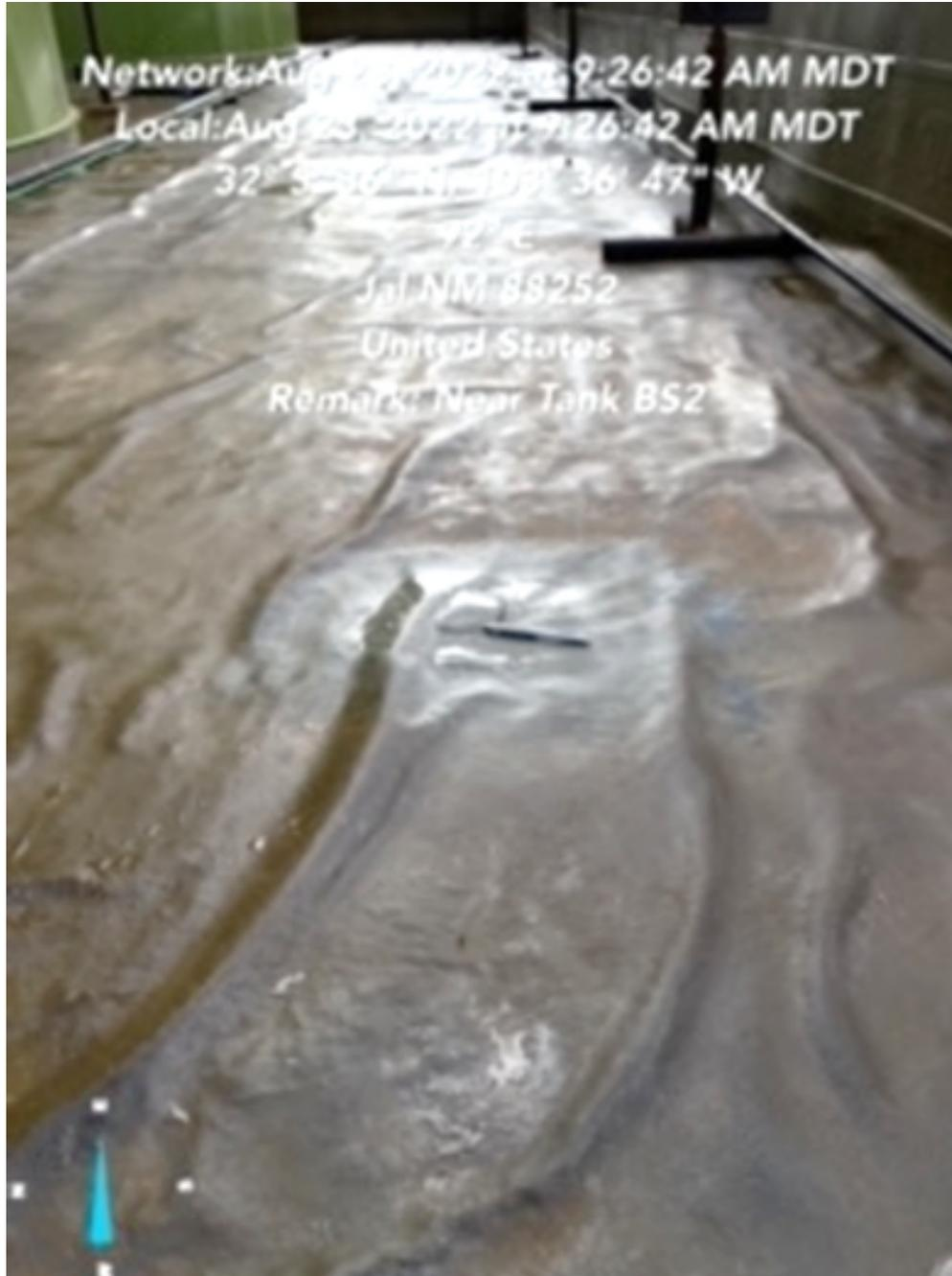
Figure 2 – Bubble in containment Northeast of tank BS2
