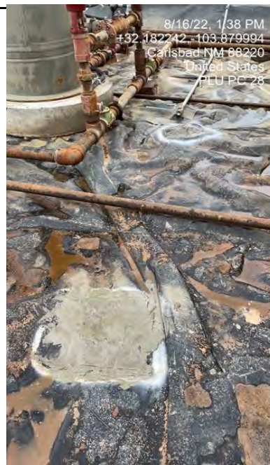
Photograph 4 Date: August 16, 2022 Description: Patched Liner
