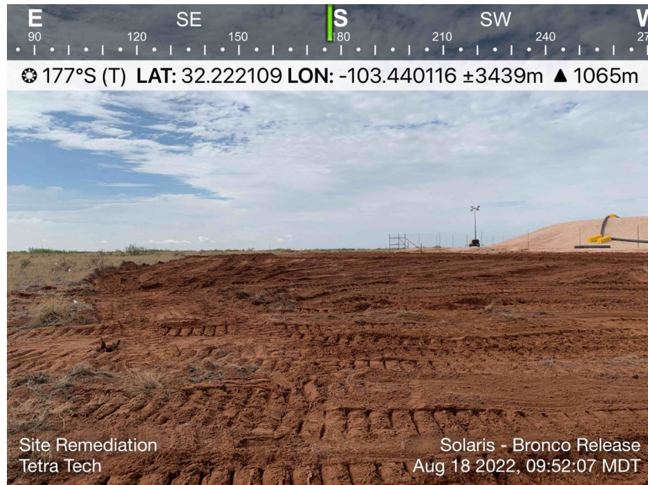
View of Initial Remediation Activities – View South
