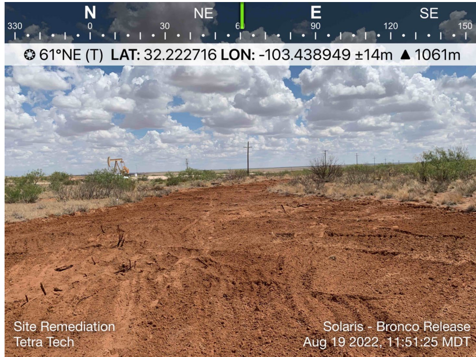
View of Initial Remediation Activities – View Northeast
