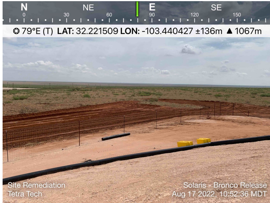
View of Initial Remediation Activities – View East
