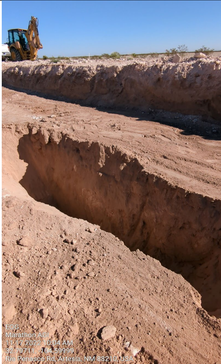
Photograph No.3 6' around excavation for backhoe Description: to reach 20'
