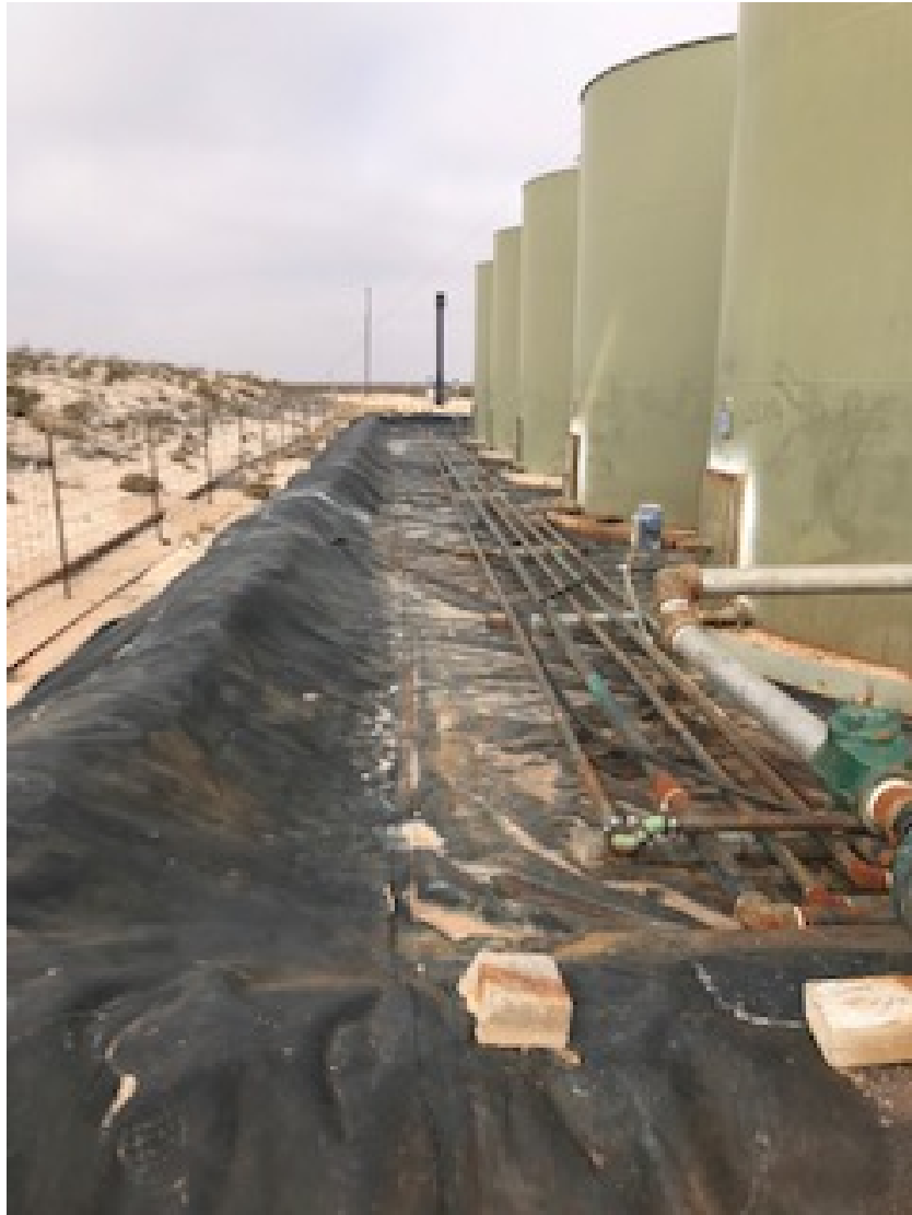
View of the lined tank battery containment.
