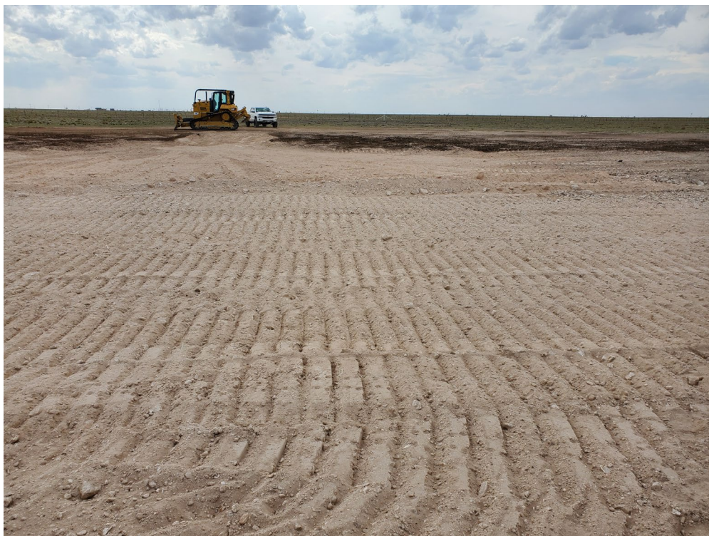
Backfilled Excavation (Caliche) Viewing West, June 25, 2021
