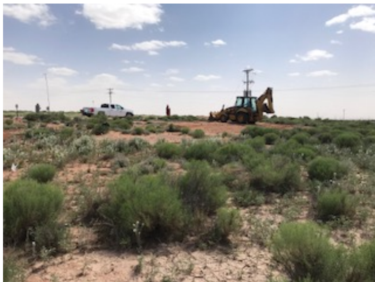
Photograph 1: View of release area facing east.
