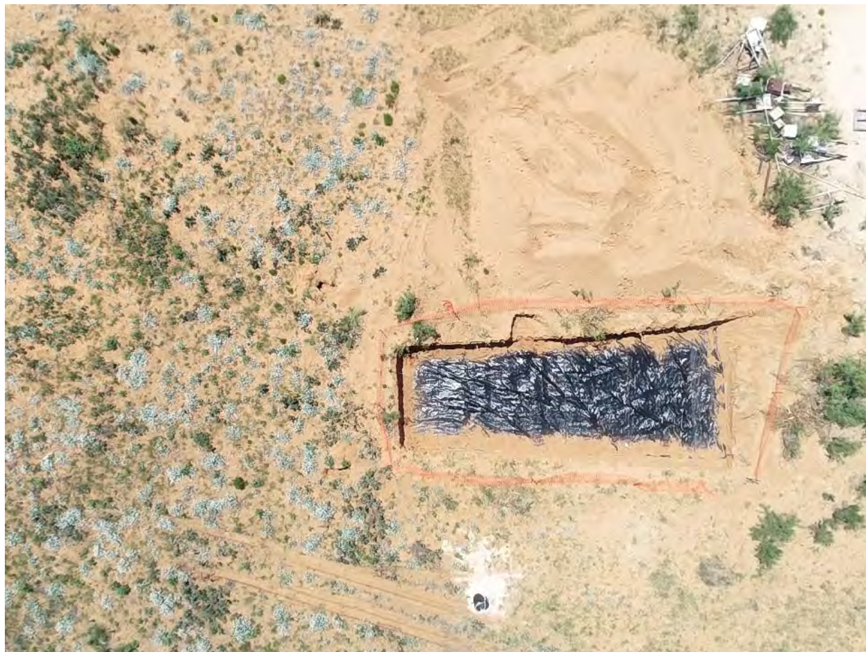
NEDU #830 Aerial with 20-mil Liner Installed, July 27, 2021
