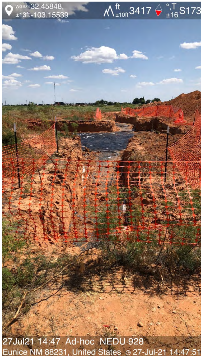
NEDU #928 with 20-mil Liner Installed, July 27, 2021
