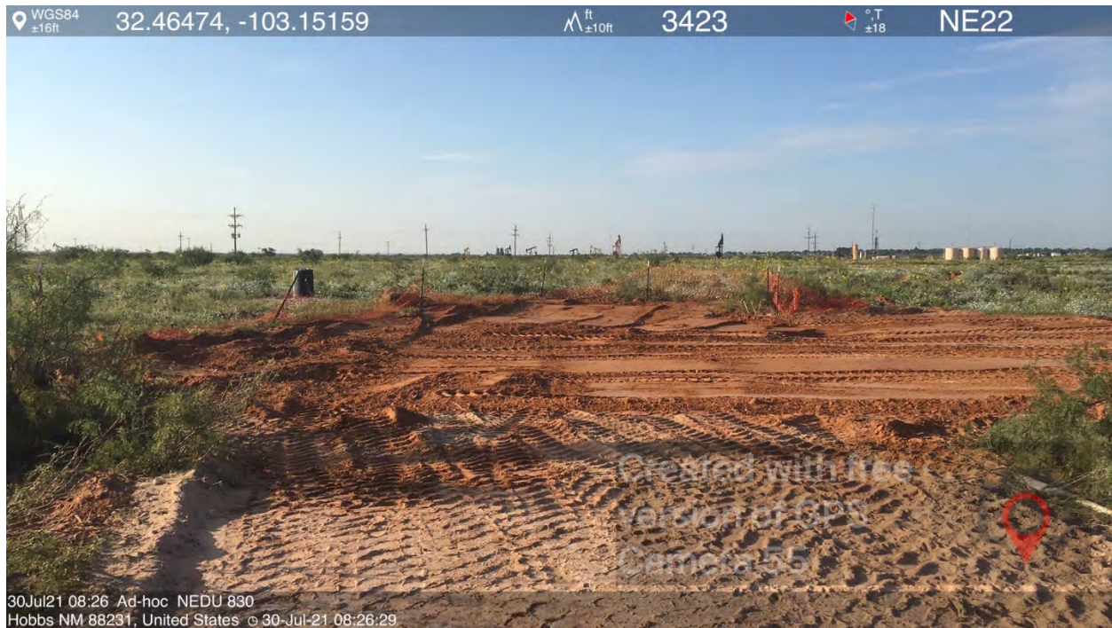
NEDU #830 Backfilled Excavation, July 30, 2021
