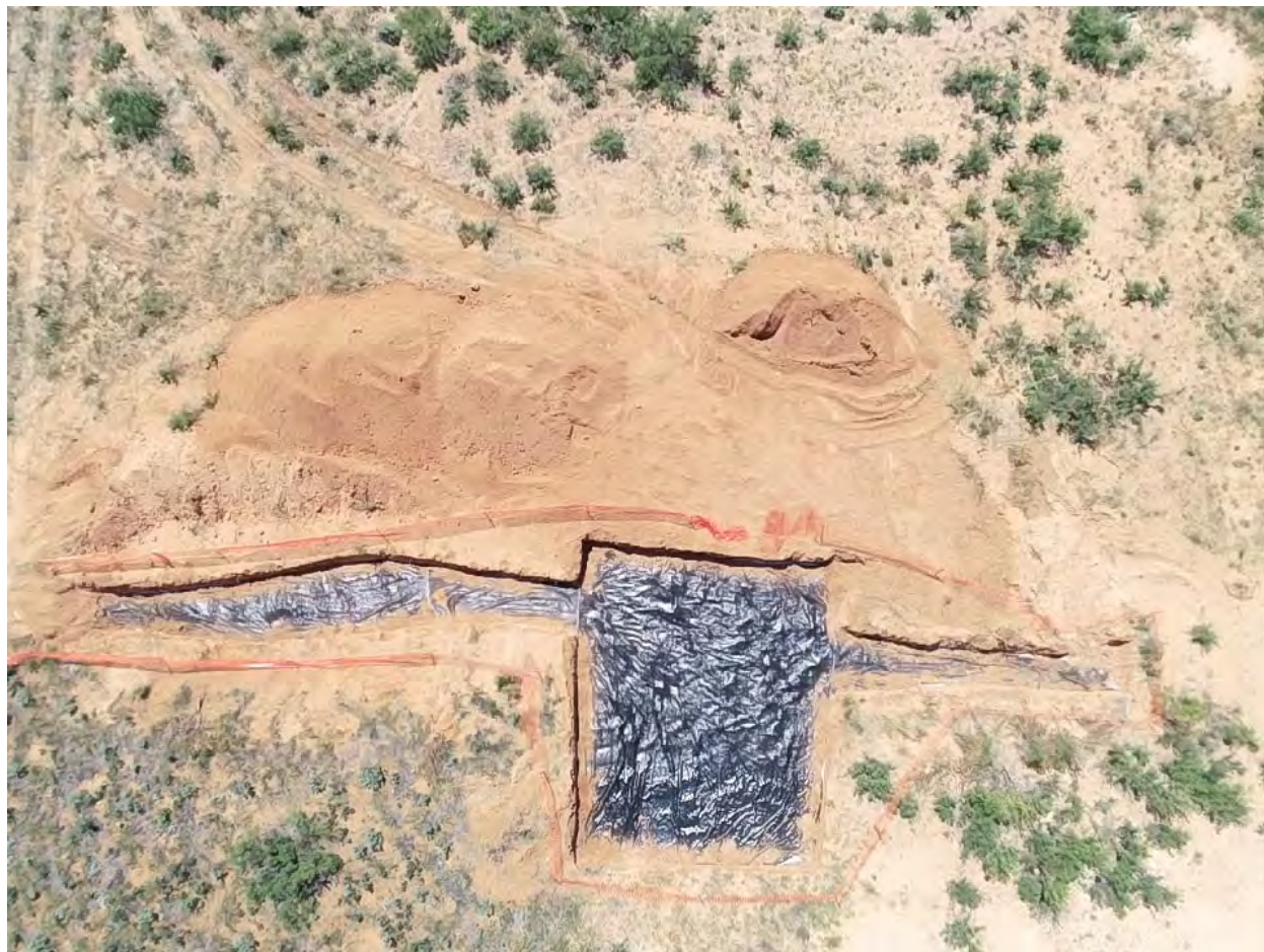
NEDU #928 Aerial with 20-mil Liner Installed, July 27, 2021
