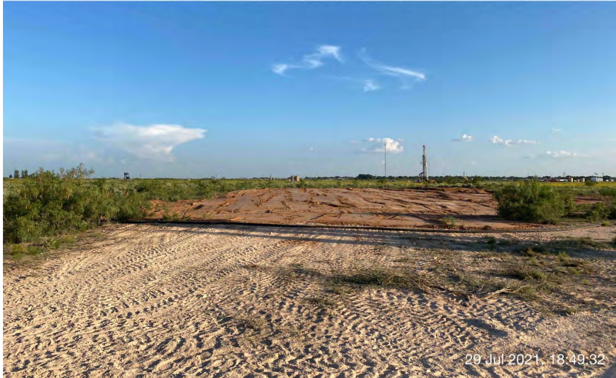
NEDU #929 Backfilled Excavation, July 29, 2021
