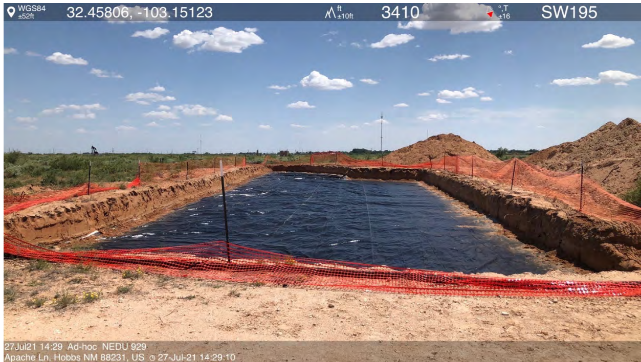
NEDU #929 with 20-mil Liner Installed, July 27, 2021
