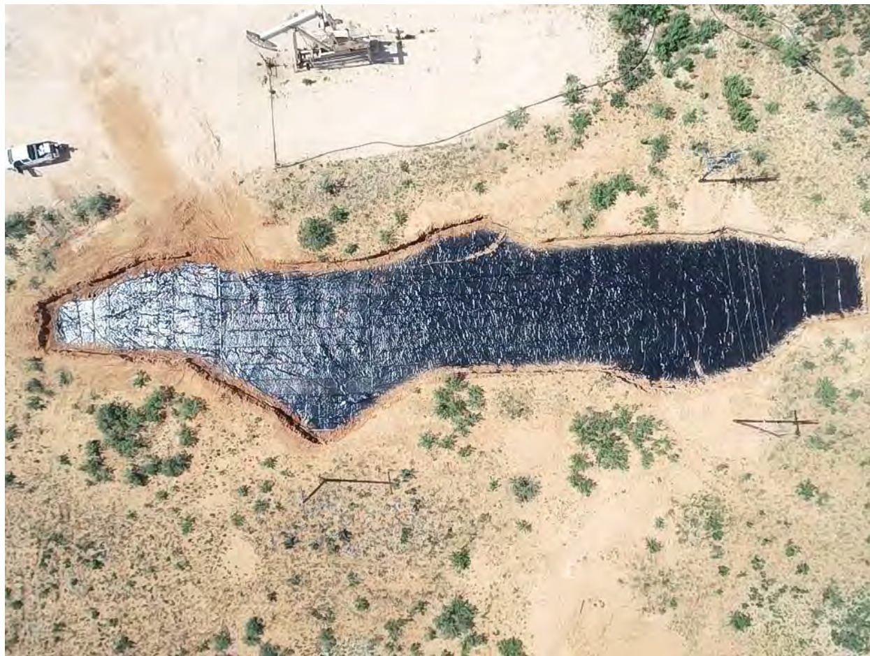
NEDU #829 Aerial with 20-mil Liner Installed, July 27, 2021
