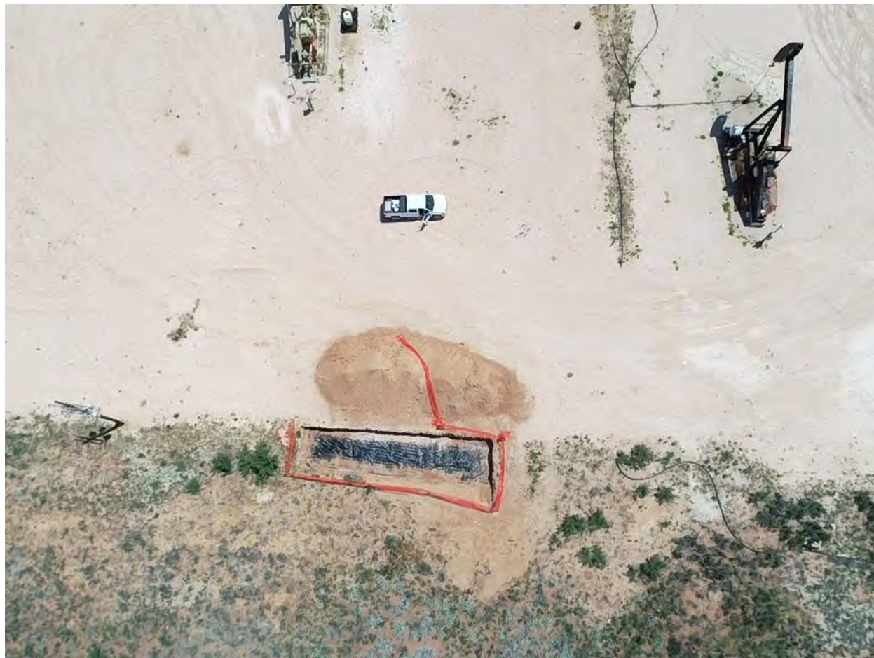
NEDU #922 Aerial with 20-mil Liner Installed, July 27, 2021
