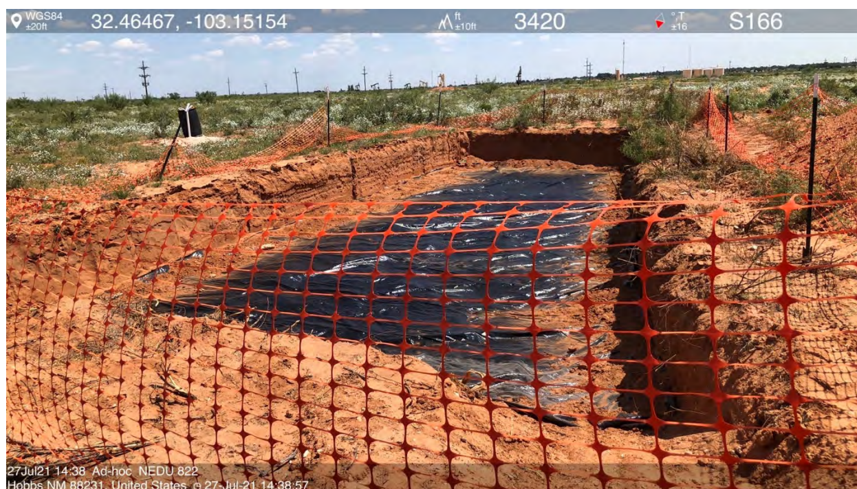
NEDU #830 with 20-mil Liner Installed, July 27, 2021
