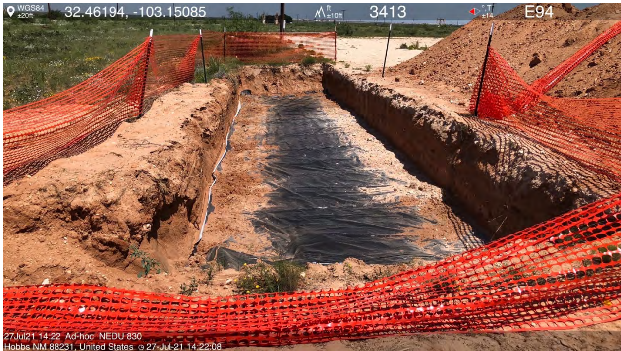
NEDU #922 with 20-mil Liner Installed, July 27, 2021
