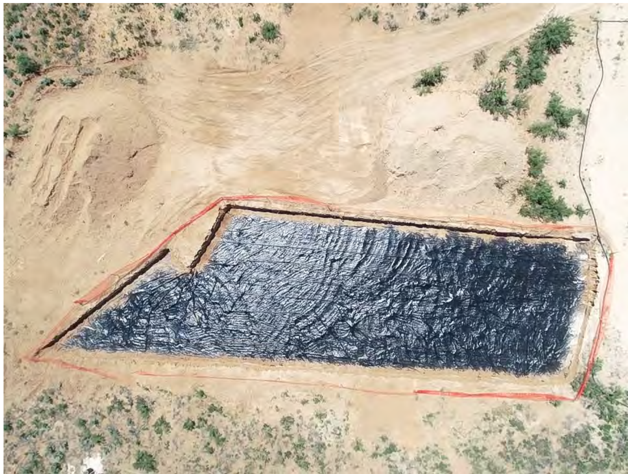
NEDU #929 Aerial with 20-mil Liner Installed, July 27, 2021
