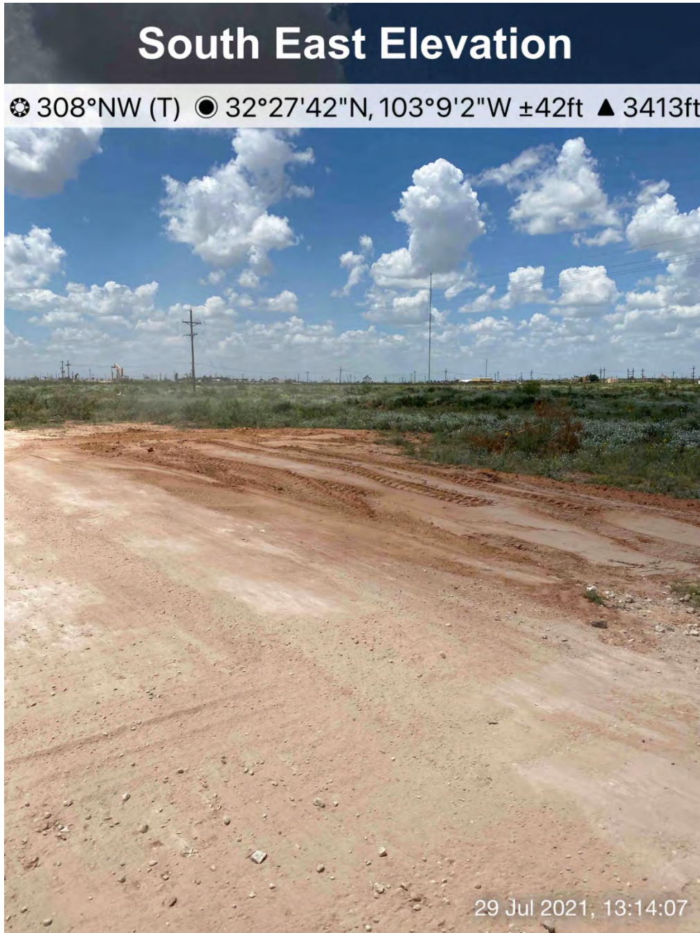
NEDU #922 Backfilled Excavation, July 29, 2021
