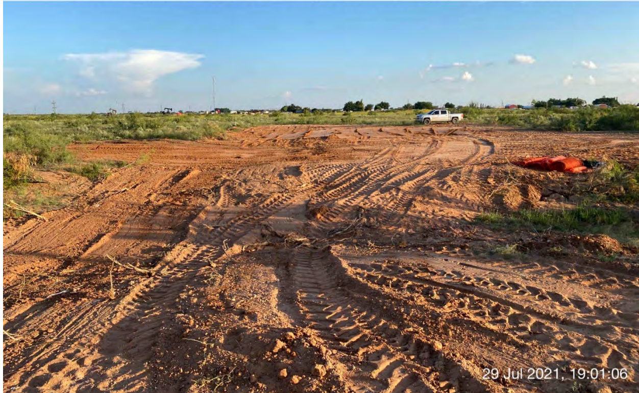
NEDU #928 Backfilled Excavation, July 29, 2021
