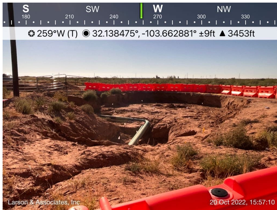
Excavated soil viewing west, October 20, 2022
