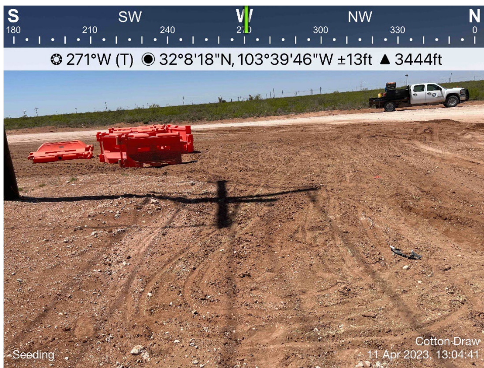
Seeded excavation viewing west, April 11, 2023
