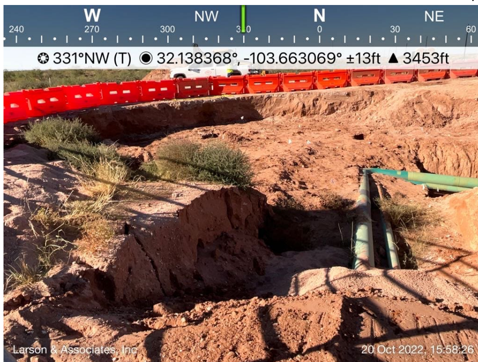
Excavated soil viewing northwest, October 20, 2022
