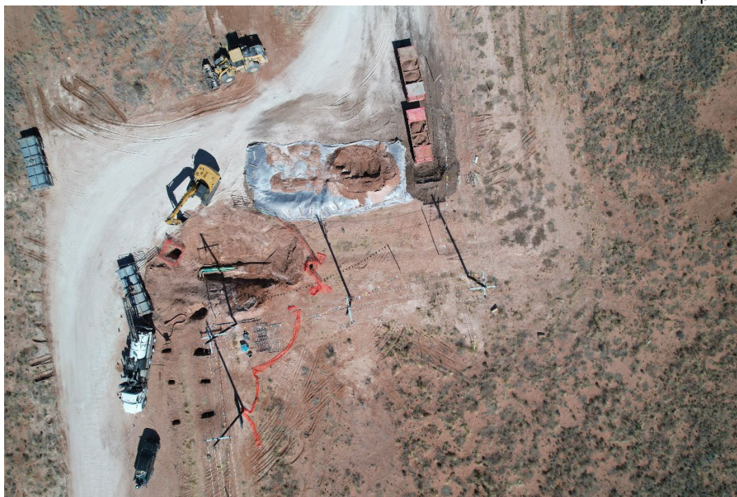
Impacted area with soil stockpiled adjacent to excavation, February 11, 2022
