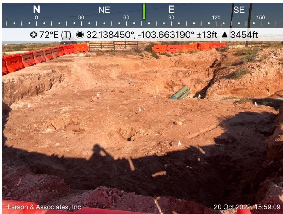
Excavated soi viewing east, October 20, 2022
