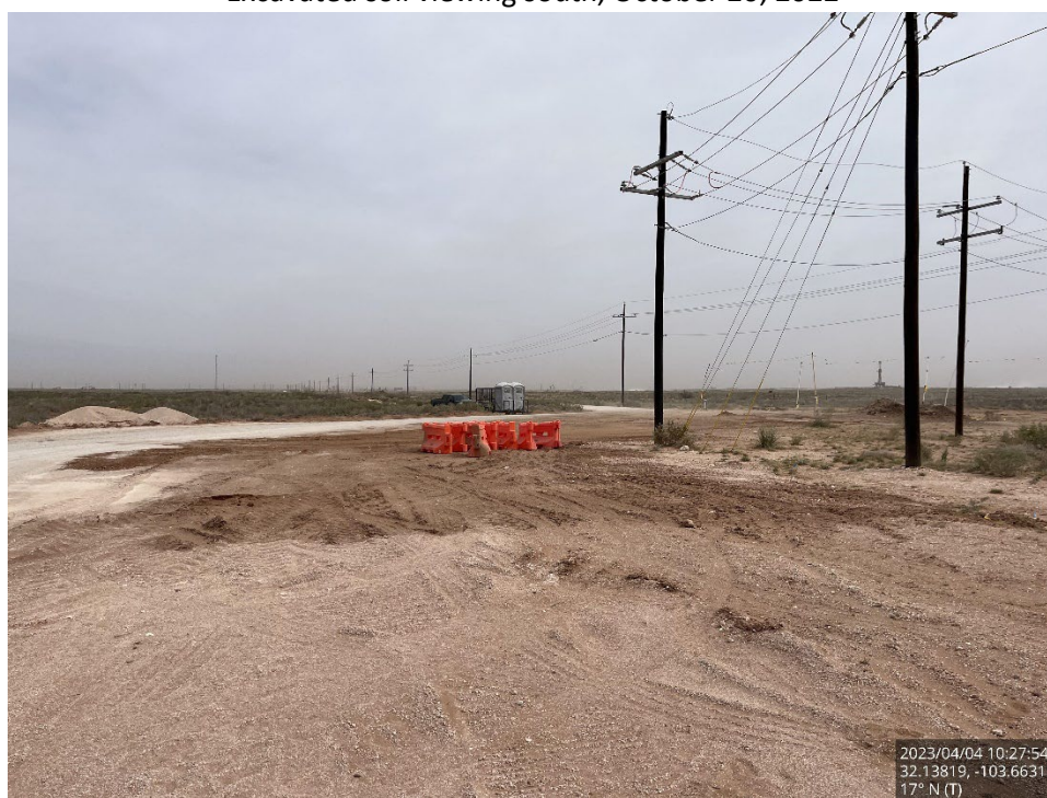
Backfilled Excavation viewing north, April 4, 2023
