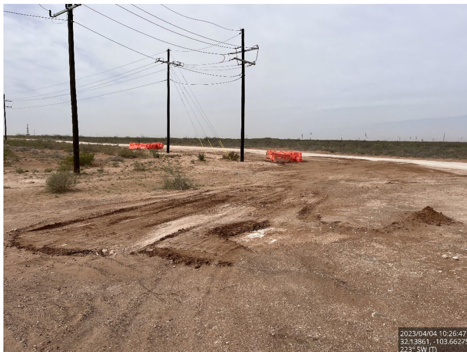
Backfilled excavation viewing southwest, April 4, 2023
