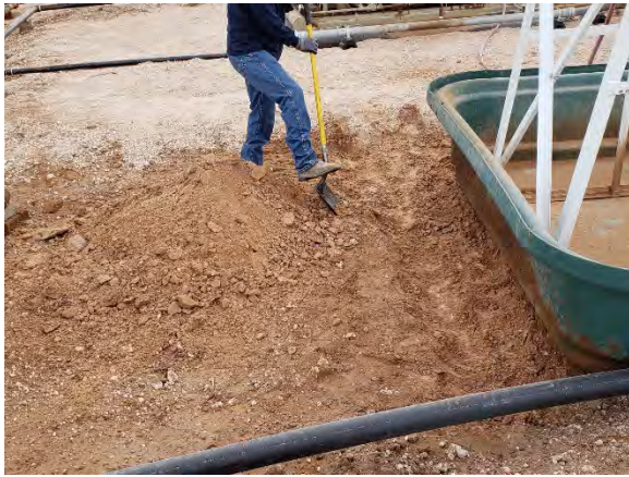
Digging up release
