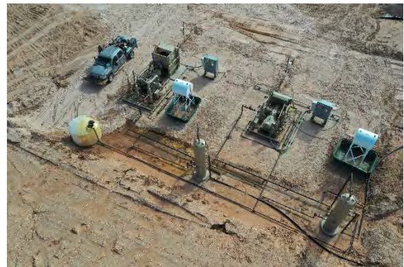
Aerial View -South View
