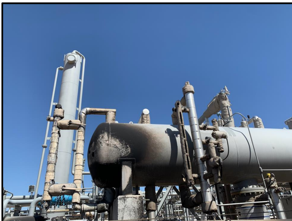
Photo of property damage to water flash tank and support
