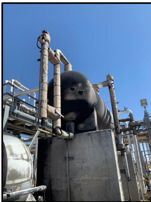
Photo of Property Damage to water flash tank and support
